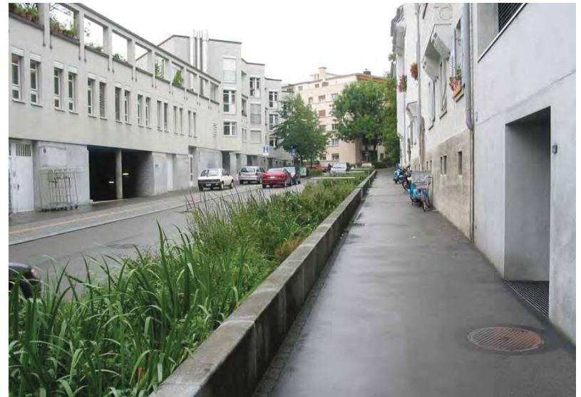
A creek daylighting project in Zurich, Switzerland protects and improves water quality, by keeping it out of the sewer, and transforms the streetscape.
