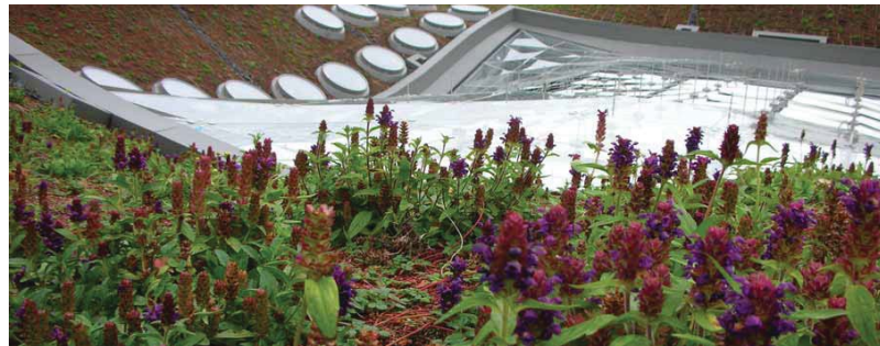
The Academy of Sciences in Golden Gate Park is targeting LEED Platinum certification and includes a 2.5 acre vegetated roof. Photo: Rana Creek - Living Architecture
