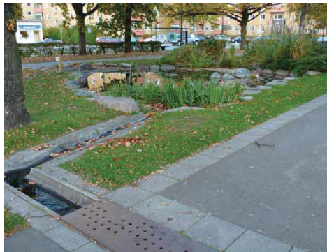
The Ekostaden residential development in Malmo, Sweden, channels all stormwater runoff through BMP treatment features such as bioswales, ponds, and wetlands as shown here. Photo: Brooke Ray Smith
