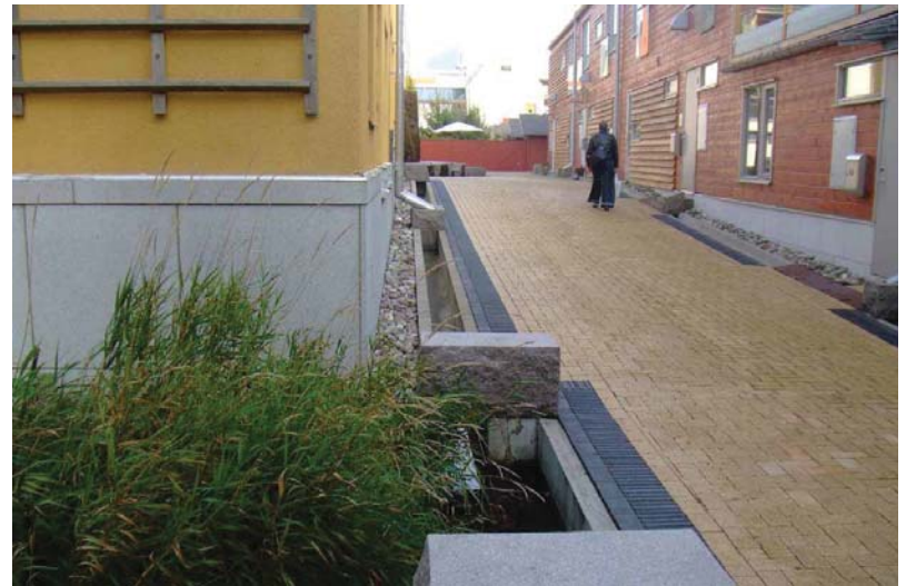
The Western Harbor, located in Malmo, Sweden, conveys and treats stormwater by implementing both parcel and block-scale surface systems that direct runoff to vegetation and ponds, which double as amenities throughout the neighborhood. Habitat value is enhanced through the use of various vegetation types. Photo: Andres Power
