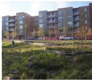
Rain gardens and a creek daylighting project are the centerpieces of open space adjacent to the Headwaters development in Portland, OR.
