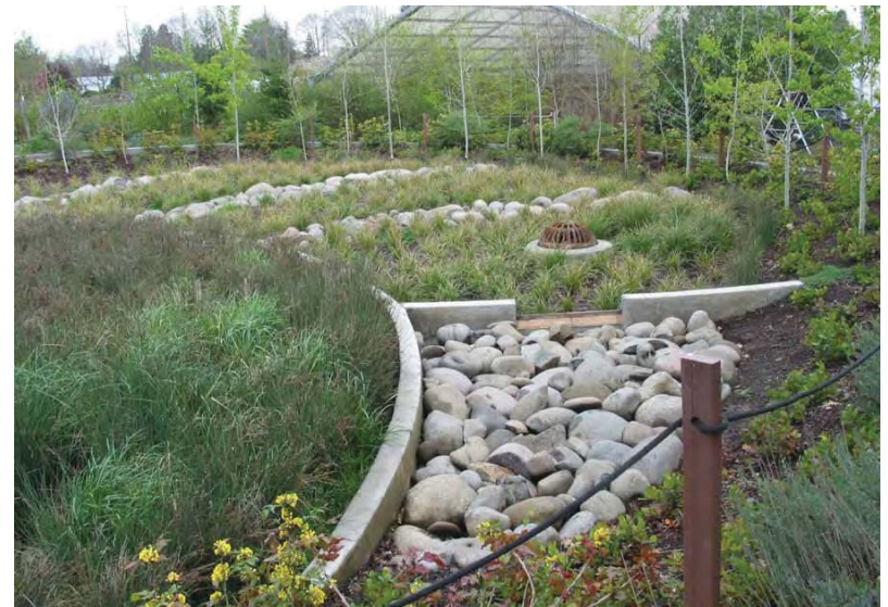
A rain garden at Glencoe Elementary in Portland, Oregon reduces stormwater flows to Portland's collection system.
