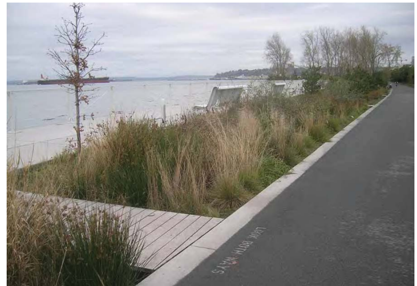
Boardwalks provide access across waterfront bioretention facilities in Seattle, WA.
