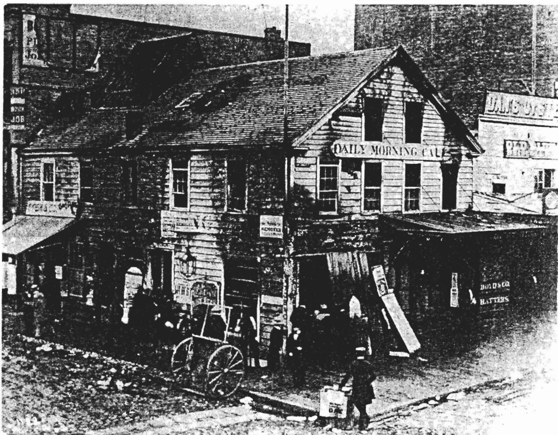
Gold Rush Streets: The corner of Montgomery and Clay in about 1859. The daguerrotypist recorded the aftermath of a fire at the Daily Morning Call , and incidentally gave us a view of San Francisco's Gold Rush street paving. Montgomery Street is cobblestoned with a flagstone pedestrian walkway to make street crossing safer and more comfortable. Clay Street appears to be brick-paved.
