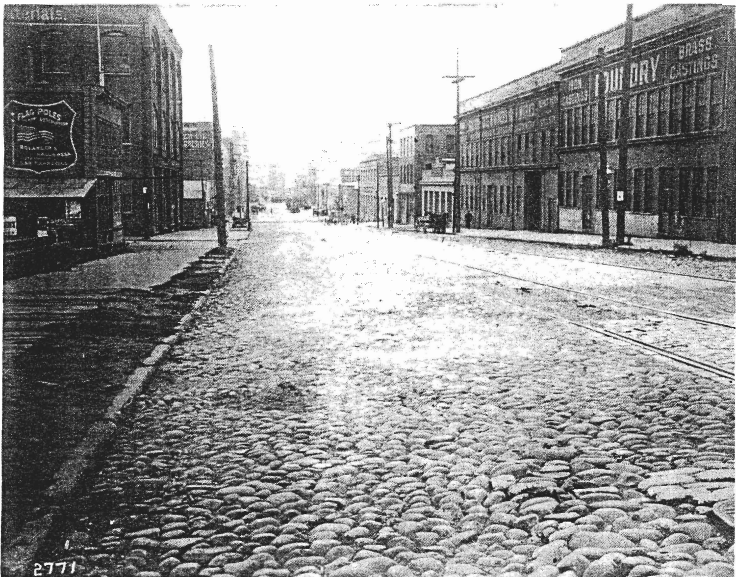
Cobblestone Paving: Looking north on First Street from Folsom in 1915. Cobblestones presented an uneven, random size that were hard on horses that still did most of the hauling. Notice that paving blocks have been laid in the center of the street car tracks. Granite street curbs like these were laid throughout the city.
