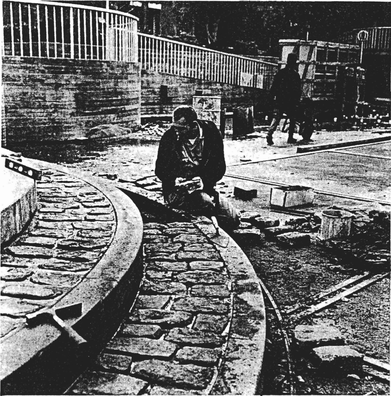
Basalt Blocks are Prized by Architects for Decorative Paving: The stone mason uses old paving blocks to make handsome steps below a fountain at Ghirardelli Square.
