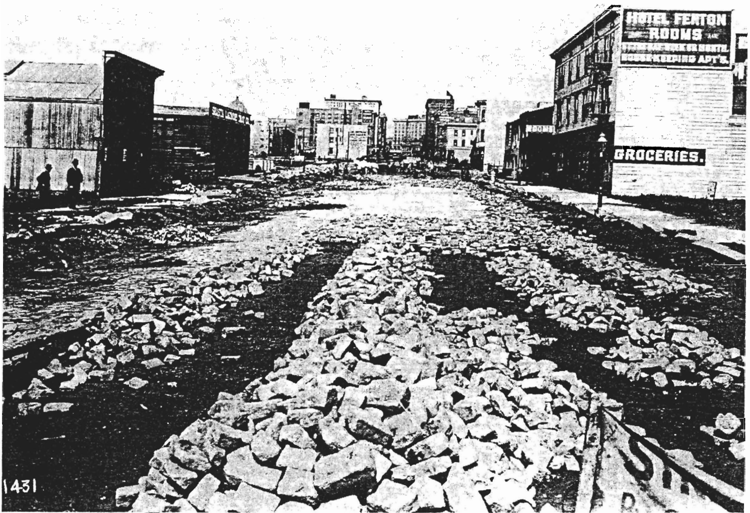
Getting Ready to Pave in 1913: The paving gang is working its way up the street. Big dray wagons have dumped the blocks to be laid on a sand foundation. It was still a gaslight era and sidewalks appear haphazard, although granite slabs are waiting to become curbs along Seventh at Folsom.
