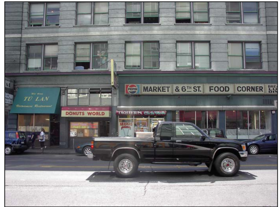
Disorganized signage distracts from creating a positive retail environment on Sixth Street.
