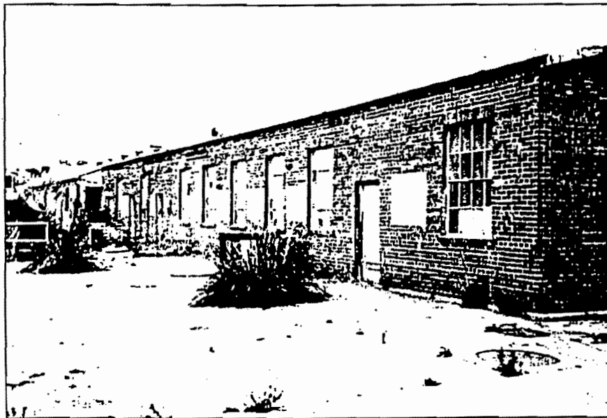
Tool and Paint Building (Building 207)
