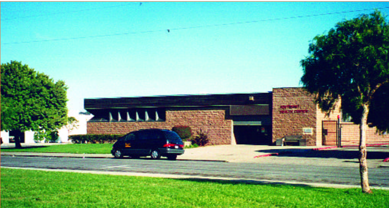
The Southeast Health Center is one of 18 primary health care facilities located throughout the City as part of the Department of Public Health's Community Health Network. Community members would like to see the facility expanded.
