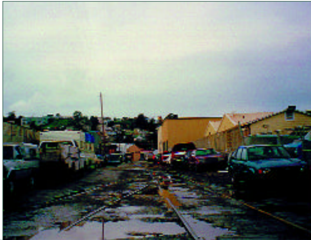
Above is an example of the need for improved street infrastructure in Bayview's Northern Industrial Area.
