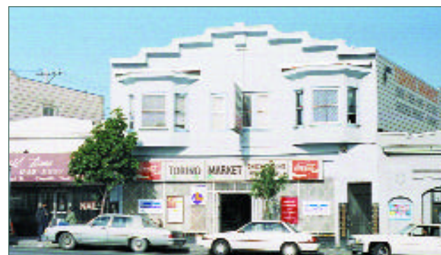
Most parking in the Third Street neighborhood commercial core will be preserved when light rail comes down Third Street.
