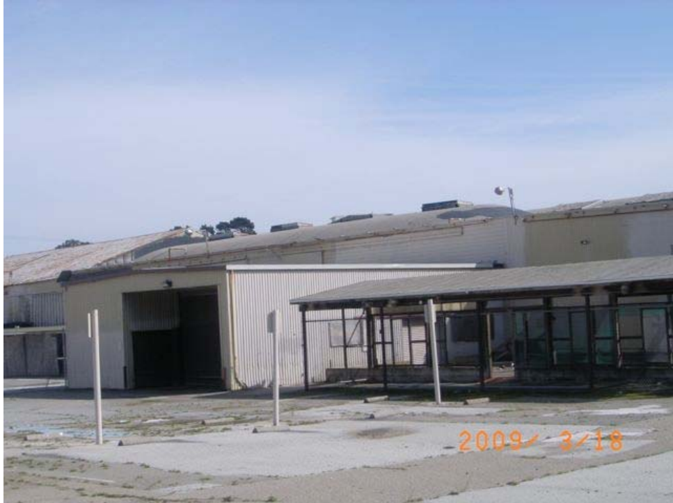
Bayshore Boulevard near Cortland Avenue: rusted roof, peeling paint, dilapidated pavement, extensive deterioration.
