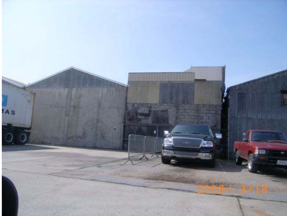
Donner Avenue between 3 rd Street and Jennings Street: damaged siding, informal and substandard construction.
