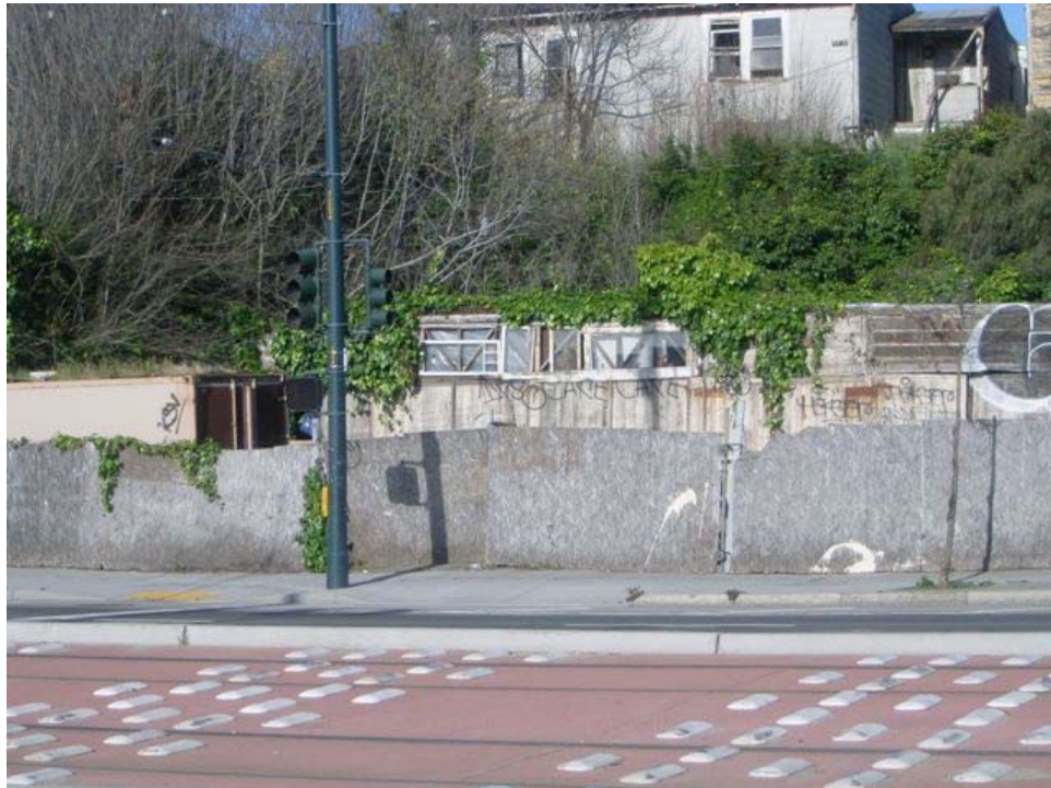
3 rd Street near Thornton Avenue: informal and substandard structure, graffiti, extensive dilapidation.
