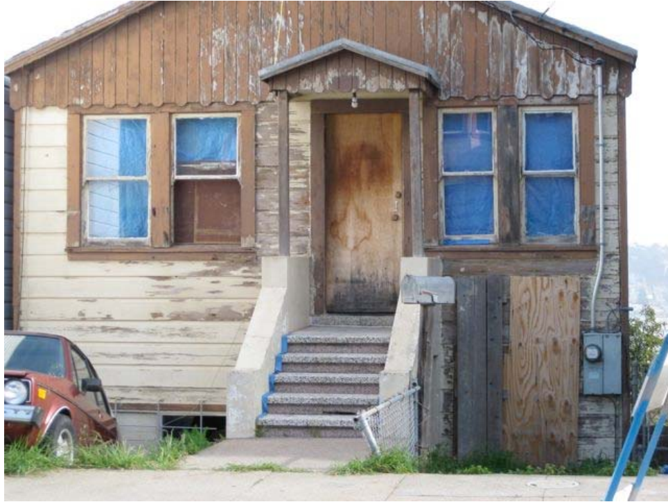
Jamestown Avenue near Ingalls Street: apparently abandoned dilapidated building, informal and substandard construction, peeling paint, broken and boarded windows, overgrown landscaping, abandoned vehicle.
