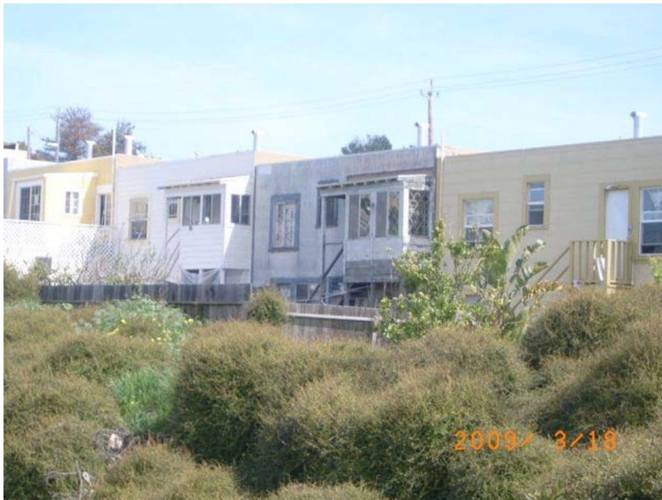
Reddy Street near Williams Avenue, rear of home: deferred maintenance, peeling paint.
