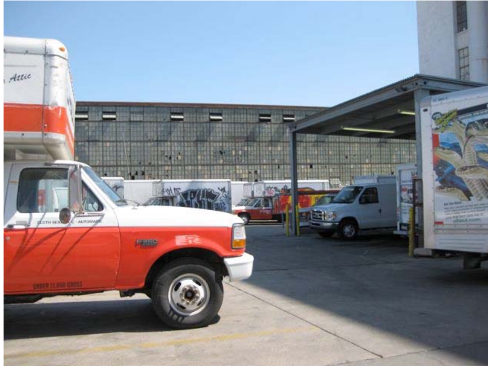
Near Bayshore Boulevard and Paul Avenue: apparently abandoned building, broken and boarded windows, graffiti.
