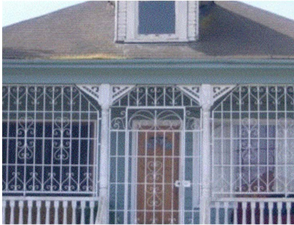
Hollister Avenue near Jennings Street (close up of above): vegetation growing from rain gutter, deteriorated attic window.
