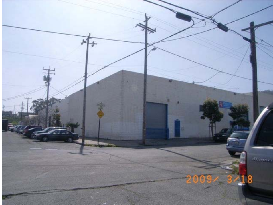
Donner Avenue near Ingalls Street: faded paint, partially reinforced masonry building.
