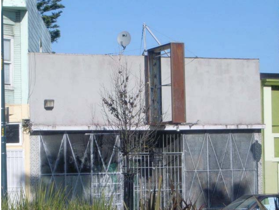
3 rd Street near LaSalle Avenue: vacant business space, dilapidated signage, water damage, peeling paint, deterioration.
