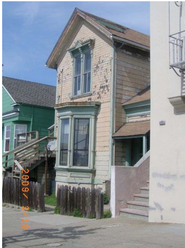
Palou Avenue near Lane Street: peeling paint, rotting wood, dilapidated roof, water damage.
