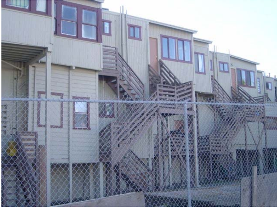
Newhall Street near LaSalle Avenue: alignment problems, substandard construction.
