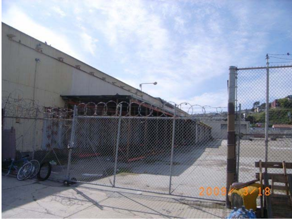
Loomis Street near Waterloo Street: vacant warehouse space, outdoor storage, trash dumping, razor wire security fencing.
