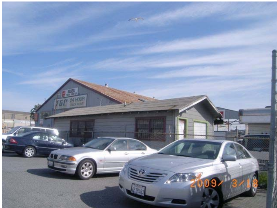
Tennessee Street near Marin Street: sagging roof, barbed wire security fence.
