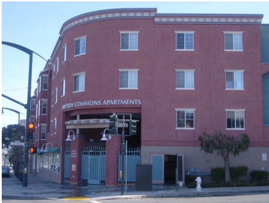
3 rd Street near LaSalle Avenue: recent housing construction.
