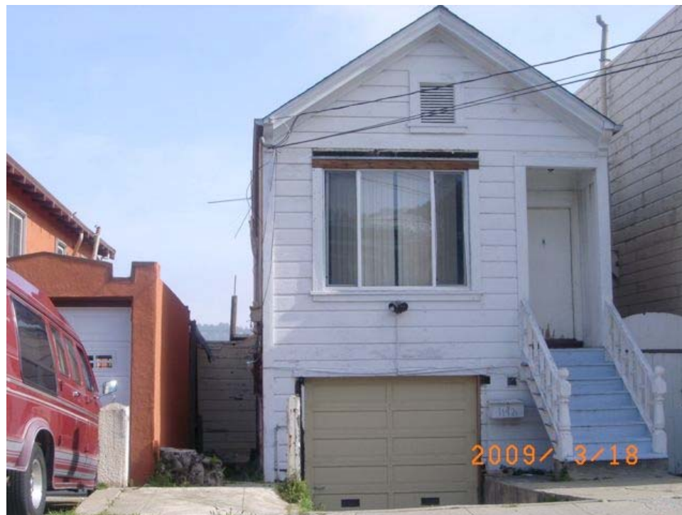
Hollister Avenue near Ingalls Street: extensive deterioration, deteriorated siding, external wiring, dilapidated door.
