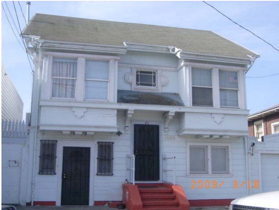
Hollister Avenue near Jennings Street: deteriorated roof, water damage, security door, window grates.
