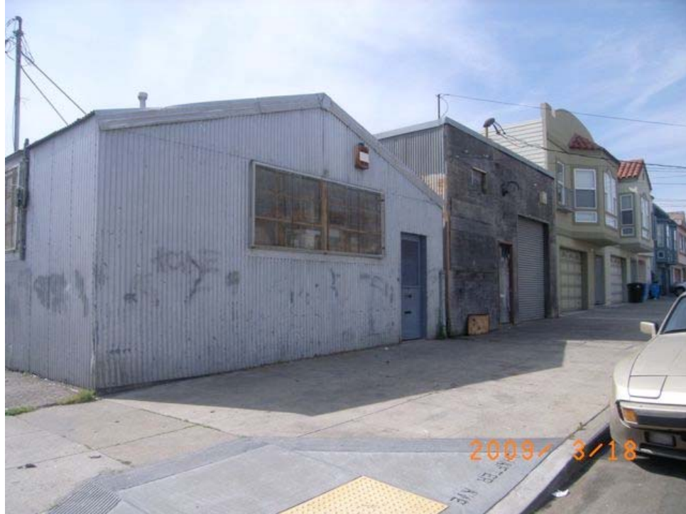
Shafter Avenue near Hawes Street: informal and substandard construction, dilapidated building, deteriorating siding, graffiti.
