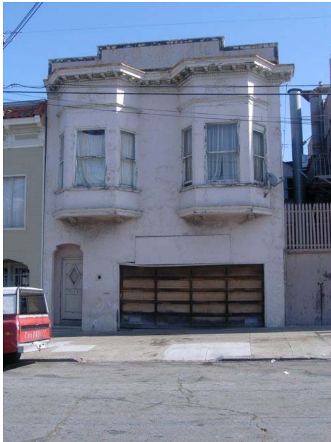
McKinnon Avenue near Newhall Street: extensive deferred maintenance, sagging floor above garage, cracked wall, dry rot, broken windows.
