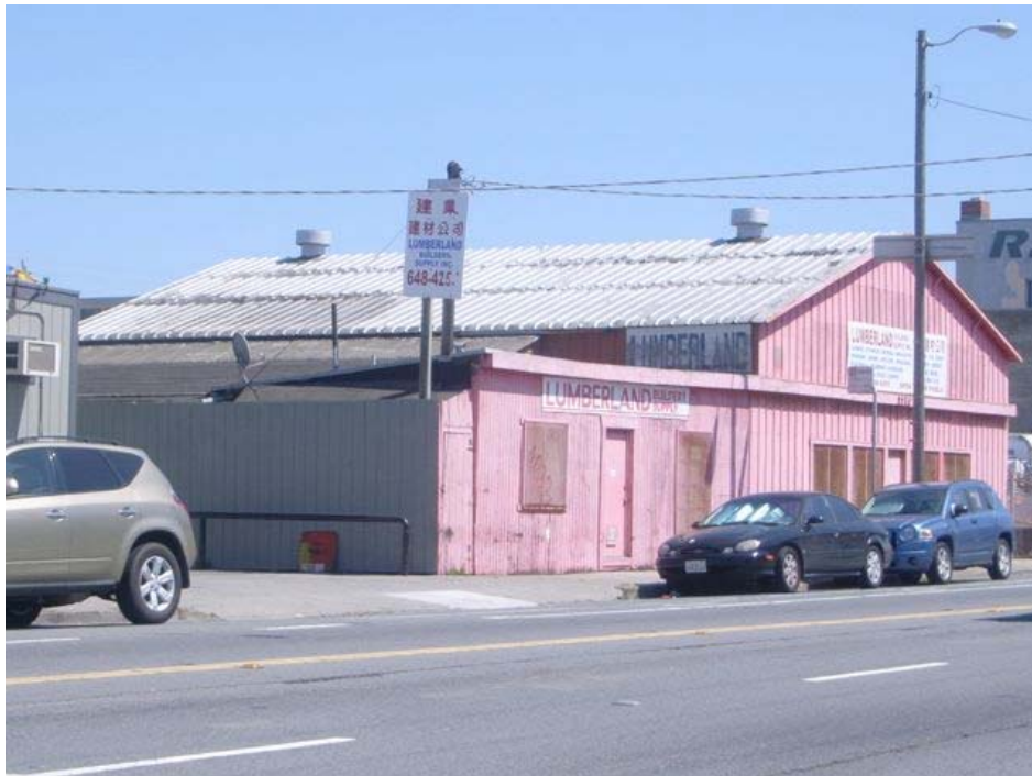
Oakdale Avenue near Barneveld Avenue: vacant business space, boarded windows, substandard and informal construction, peeling paint, graffiti, deteriorating and sagging roof.
