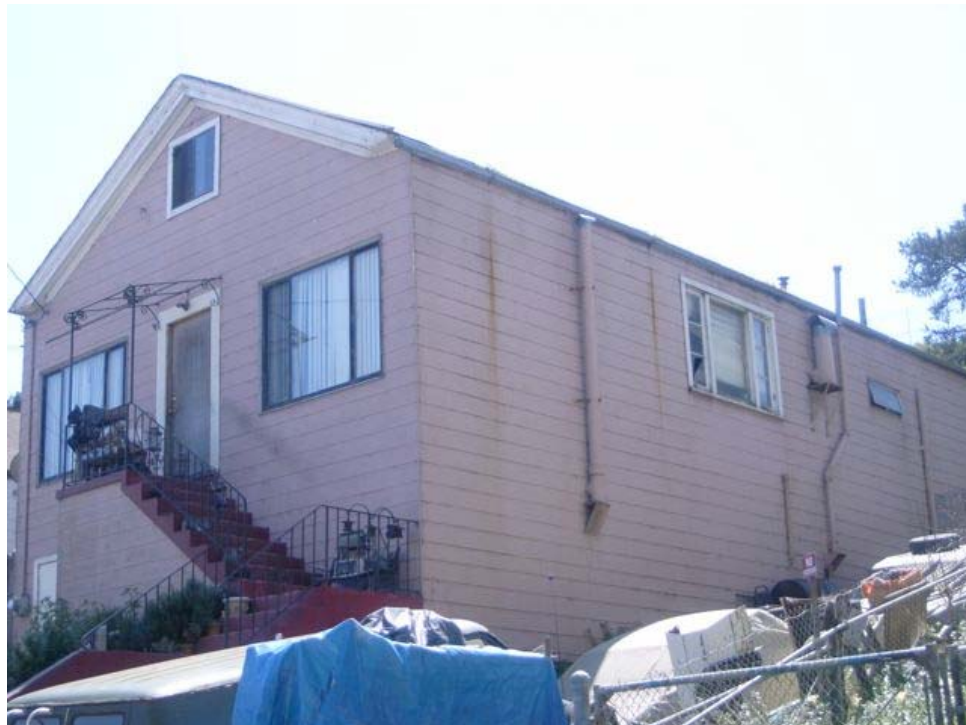
Revere Avenue near I-280: deferred maintenance, water damage on siding, possible dry rot.
