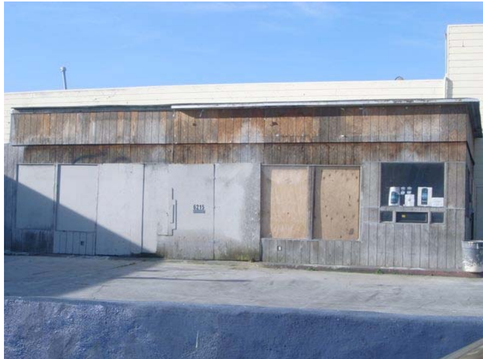
Gilman Avenue near 3 rd Street: informal and substandard construction, boarded windows, deferred maintenance, missing or deteriorated eaves.
