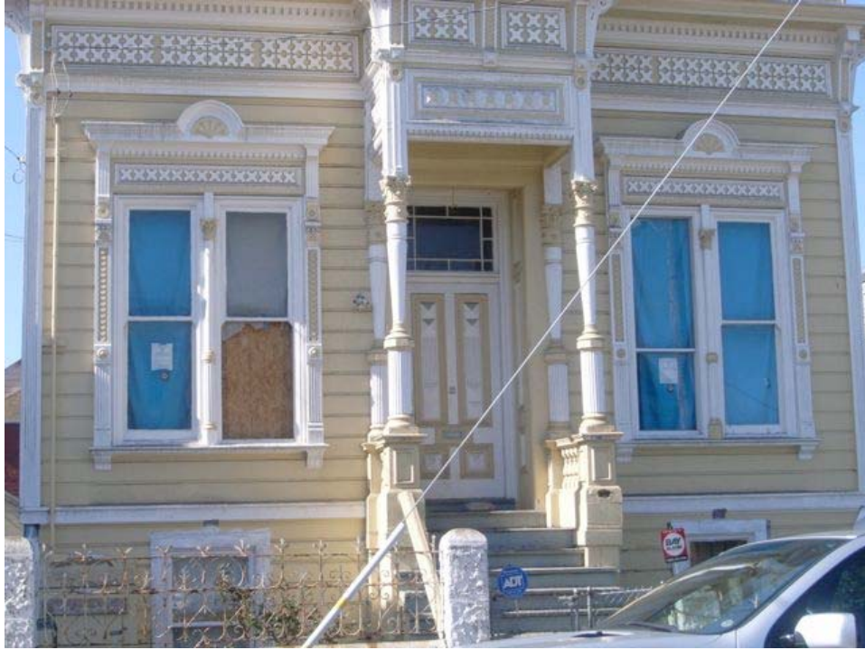
Jerrold Avenue near 3 rd Street: broken and boarded windows, peeling paint, extensive deterioration.
