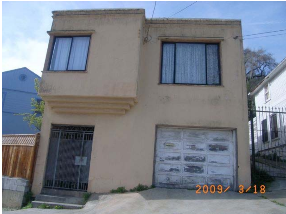
Ignacio Avenue near Ingerson Avenue: cracked wall, peeling paint, water damage, extensive deterioration.
