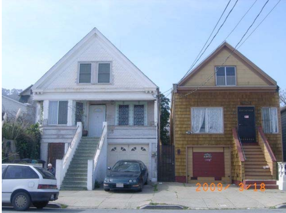
Gilman Avenue near Ingalls Street: deferred maintenance, dry rot, water damage, peeling paint.
