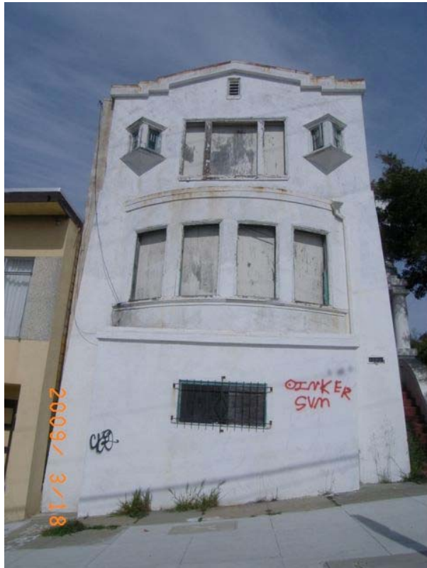
Newcomb Avenue near Lane Street: dilapidated and abandoned house, boarded windows, water damage, graffiti, external wiring.
