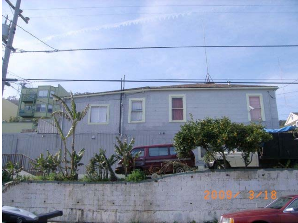
Ingerson Avenue near Hawes Street: aging retaining wall supporting driveway, residence with faded paint, water damage, security camera.
