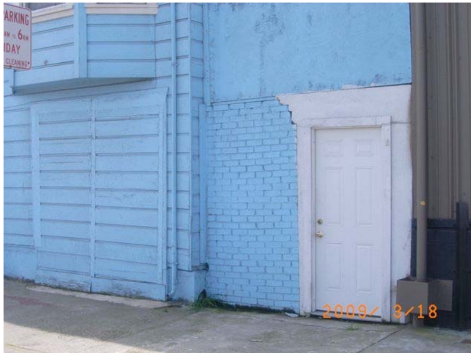
Egbert Avenue near Ingalls Street: informal and substandard construction, water damage, alignment problems.
