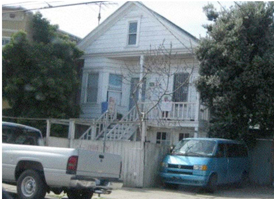
Hollister Avenue near Jennings Street: deteriorating fence, security door, security grates on windows.
