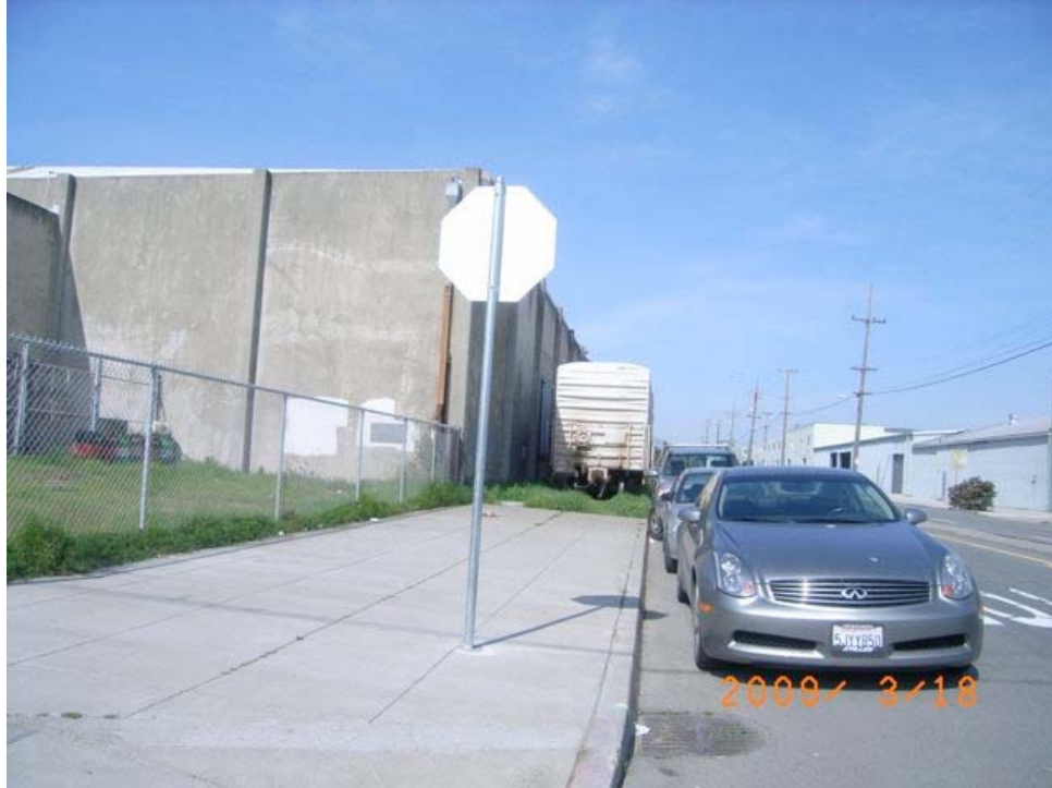
Carroll Avenue near Jennings Street: cracked concrete structure, graffiti removal, abandoned train car in public right-of-way, unpaved sidewalk.
