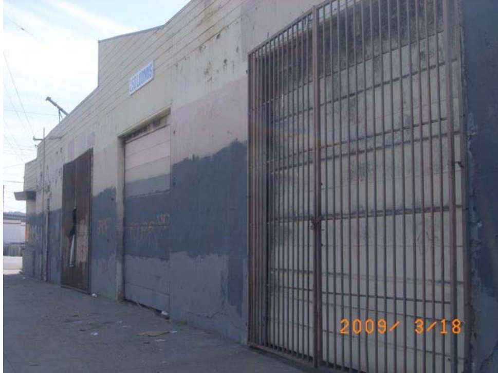
Loomis Street near Industrial Street: vacant and dilapidated building, large crack on the wall, deteriorated siding, graffiti, peeling paint, security grate.
