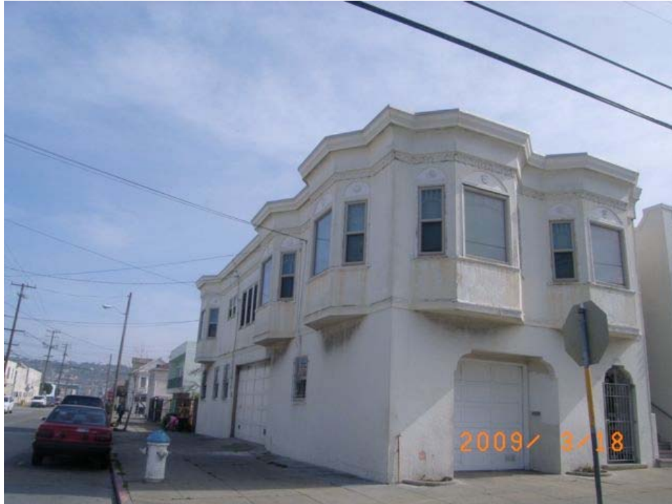
Gilman Avenue near Jennings Street: cracked wall, building deterioration, peeling paint, and water damage.
