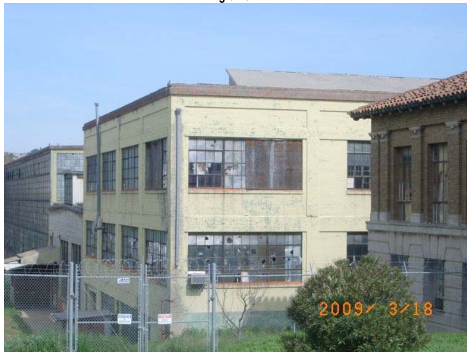
Paul Avenue and Wheat Street: apparently abandoned building, broken windows, peeling paint, extensive deterioration, barbed-wire fence.
