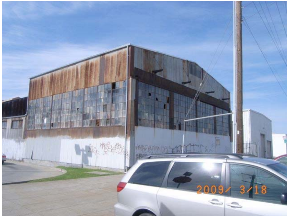
Bayshore Boulevard near Costa Street: extensive deterioration, broken windows, deteriorated siding, graffiti, eroded foundation.
