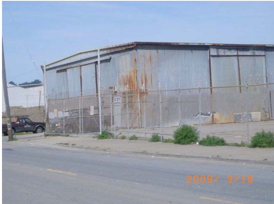
Loomis Street near Waterloo Street: rusted and dilapidated roofing and siding, razor wire security fencing.
