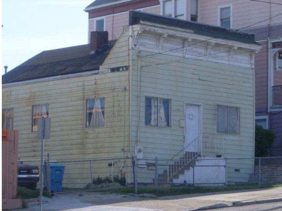
3 rd Street near Jerrold Avenue: extensive deterioration, peeling paint, water damage, deteriorated roof and chimney.
