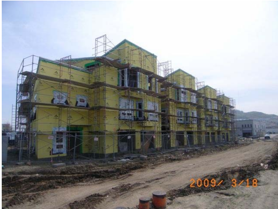
Armstrong Avenue near Mendell Street: new residential construction.
