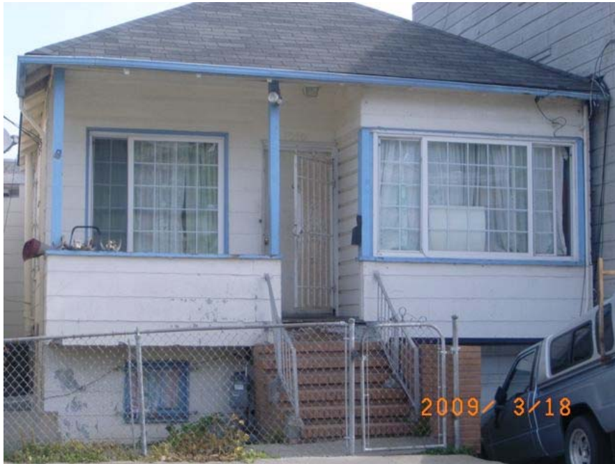
Hollister Avenue near Hawes Street: deterioration, peeling/cracking siding, peeling paint, external wiring.
