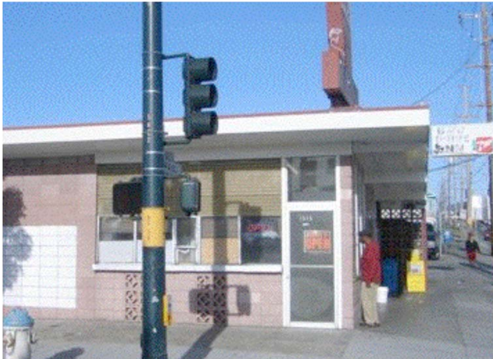
3 rd Street at Paul Avenue: deferred maintenance, graffiti on both signs, deteriorated signage.
