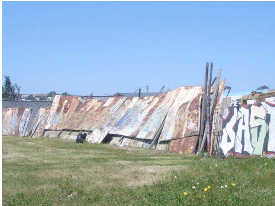
Wallace Avenue near Hawes Street: informal and substandard construction, graffiti, dilapidated fencing.
