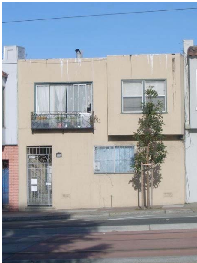
3 rd Street near Yosemite Avenue: deteriorated building, exposed wiring, water damage, cracked wall.
