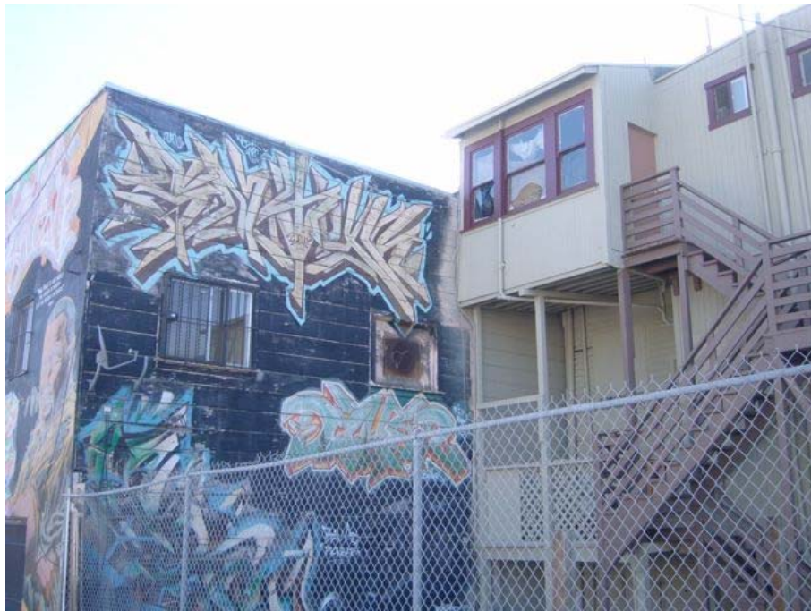
Newhall Street near Lasalle Avenue: alignment problems, substandard construction, broken and boarded windows.
