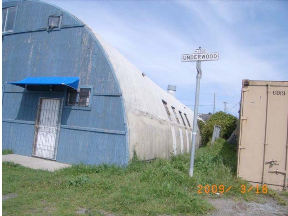
Underwood Avenue near Hawes Street: peeling paint; deteriorating siding, roofing and fencing; lack of sidewalk.
