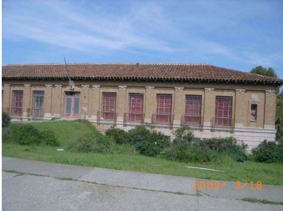
Paul Avenue near Wheat Street: long-vacant building with shuttered windows.
