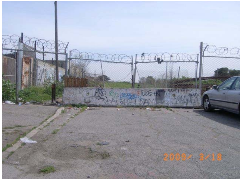
Wallace Avenue near Ingalls Street: graffiti, trash accumulation, blocked right of way.
