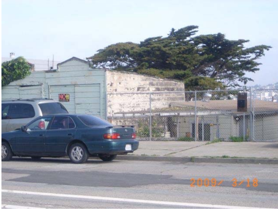
Jamestown Avenue near Hawes Street: peeling paint, water damage, alignment problems, extensive deterioration.
