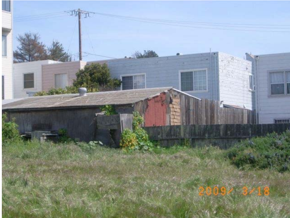
Reddy Street near Williams Avenue, rear of property: informal and substandard construction, peeling paint, deteriorated roofing.
