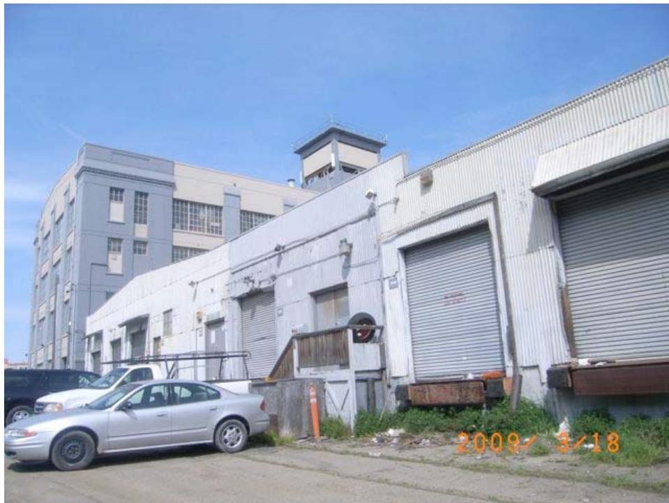
Armstrong Avenue and Mendell Street: trash accumulation, peeling paint.
