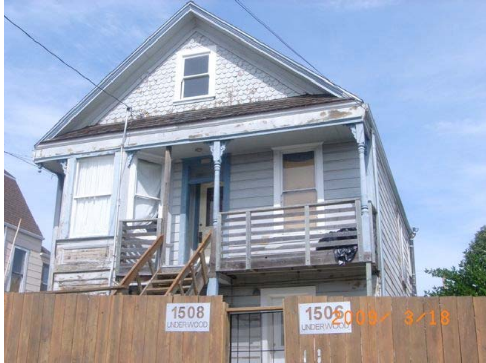
Underwood Avenue near Keith Street: deterioration, informal and substandard construction, peeling paint, evidence of dry rot.
