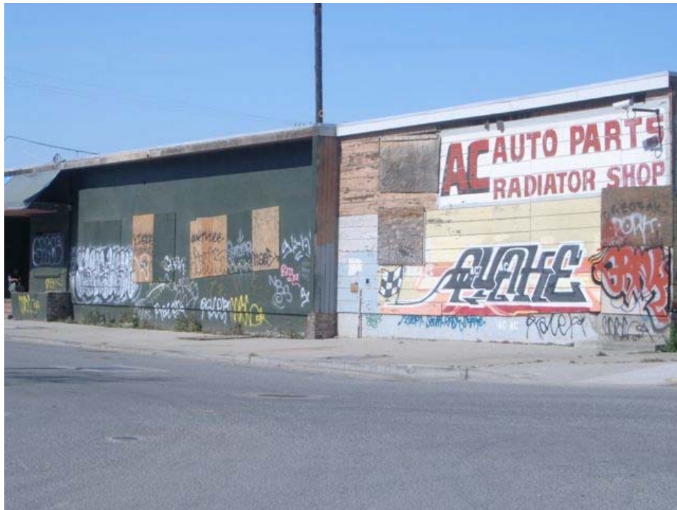
Davidson Avenue near Rankin Street: graffiti, informal and substandard construction, boarded windows.
