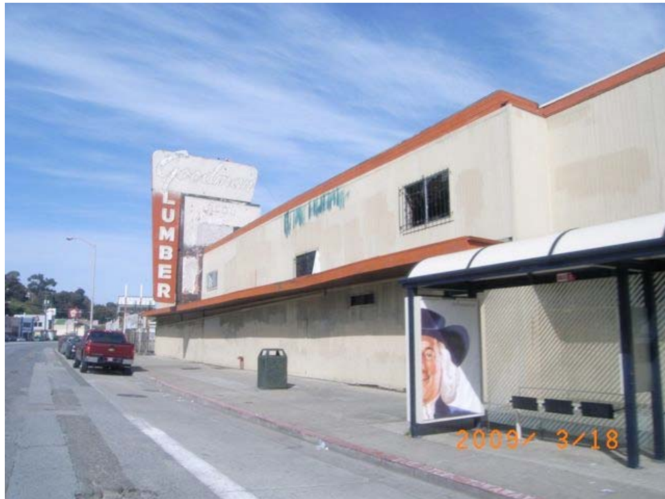
Bayshore Boulevard near Cortland Avenue: vacant and dilapidated commercial building, graffiti, sagging awning, security grates.
