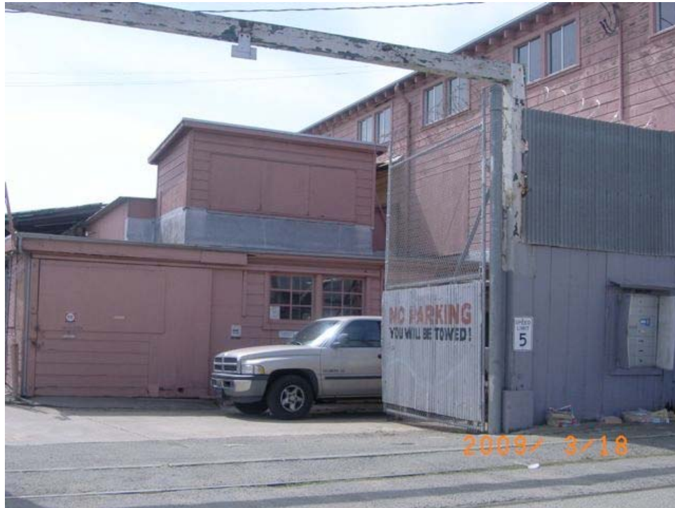
Egbert Avenue near Newhall Street: peeling paint; evidence of water damage; trash accumulation; lack of sidewalk, curb or gutter; and abandoned rail lines.
