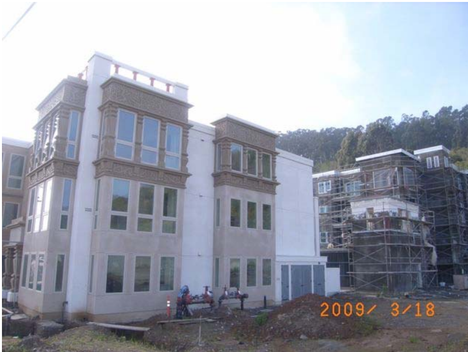
Jamestown Avenue near Redondo Street: interrupted residential development.
