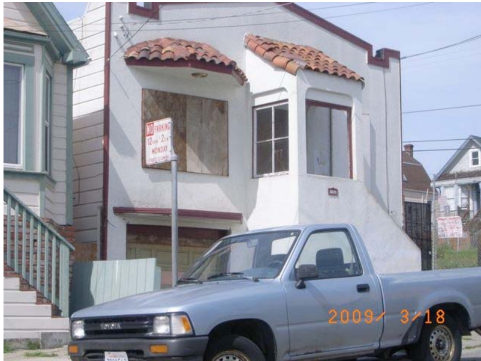
Keith Street near Underwood Avenue: vacant property with no broker information, boarded windows, roof deterioration, evidence of dry rot.
