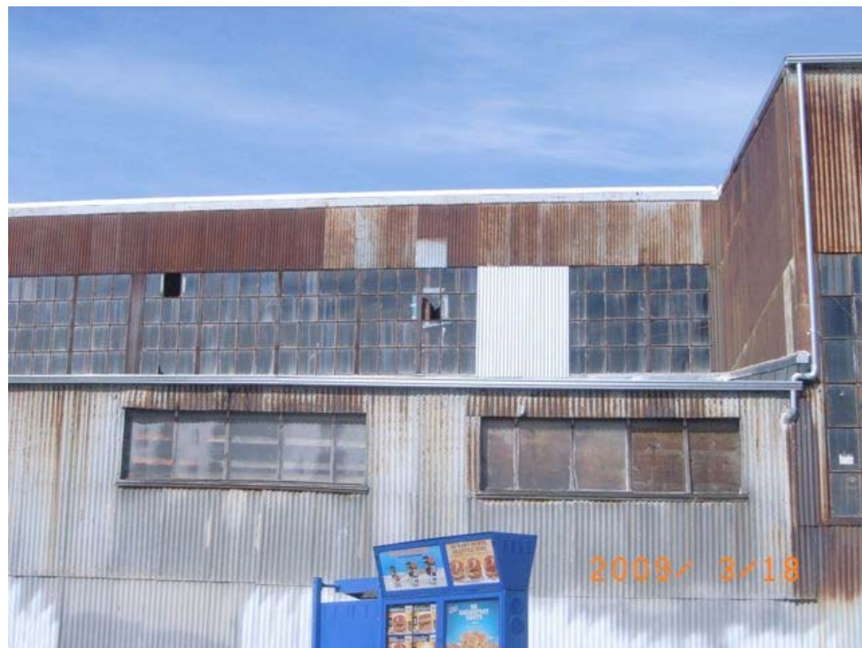
Bayshore Boulevard near Costa Street: extensive deterioration, broken windows, informal and substandard construction, deteriorated siding, graffiti.
