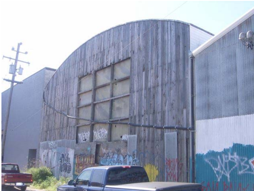
Newcomb Avenue near Toland Street: dilapidated building, graffiti, informal and substandard construction, broken windows.
