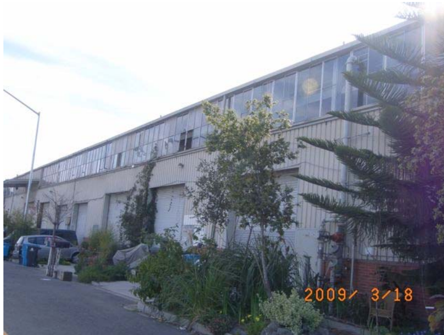
Illinois Street near Marin Street: mailboxes indicating possible residential use of industrial building.
