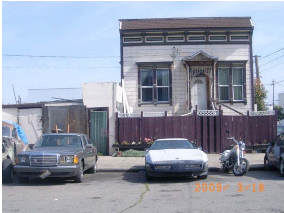
Egbert Avenue near Ingalls Street: informal and substandard construction, water damage, outdoor storage.
