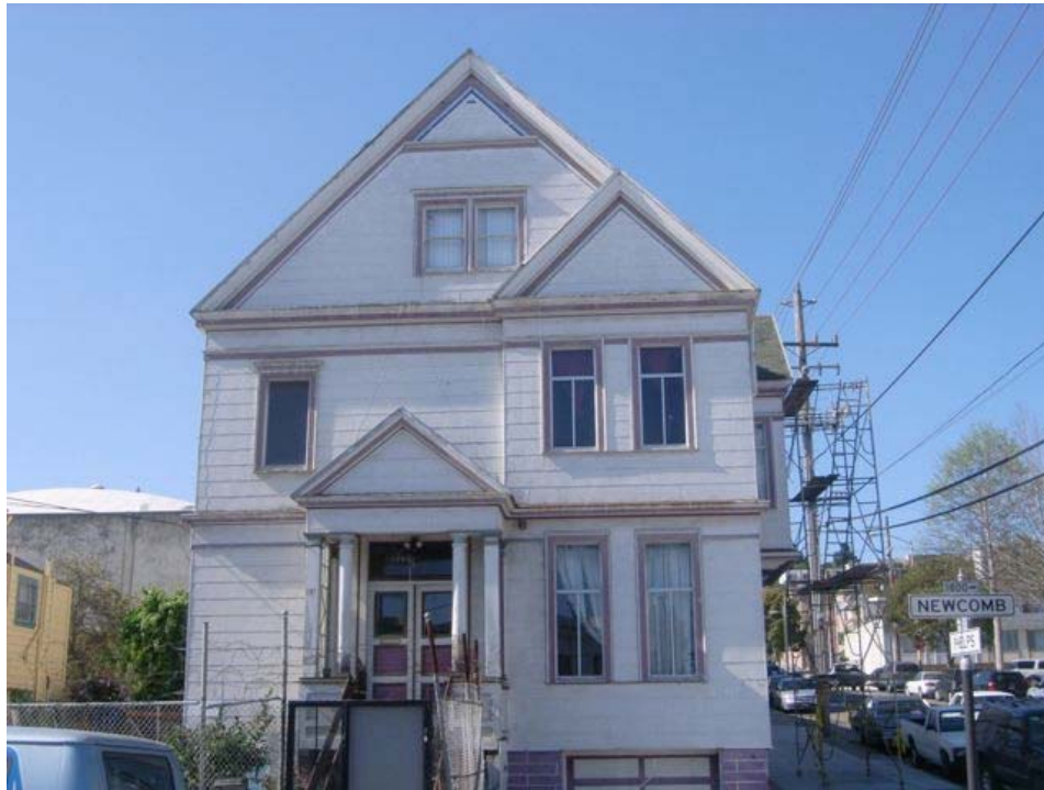
Newcomb Avenue at Phelps Street: external wiring, substandard and informal construction, peeling paint.
