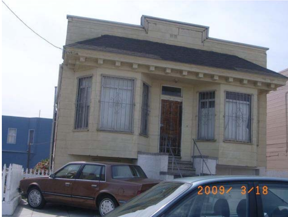
Underwood Avenue at Jennings Street: chipped/cracked siding, security grates and door, evidence of dry rot, deferred maintenance.
