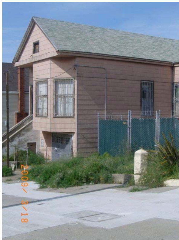
Newcomb Avenue near Lane Street: water damage, faded paint, deteriorated fencing, overgrown landscaping.
