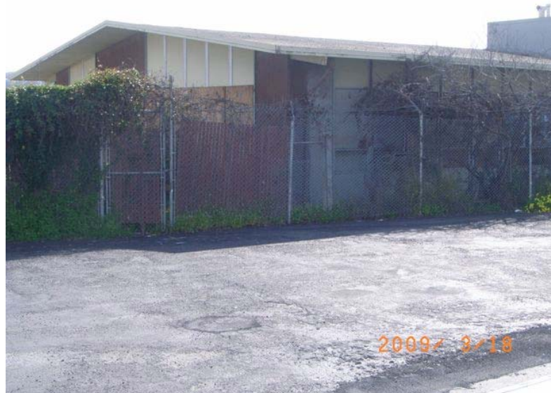
Cesar Chavez Street near I-280: vacant building, boarded windows, overgrown landscaping, extensive dilapidation.
