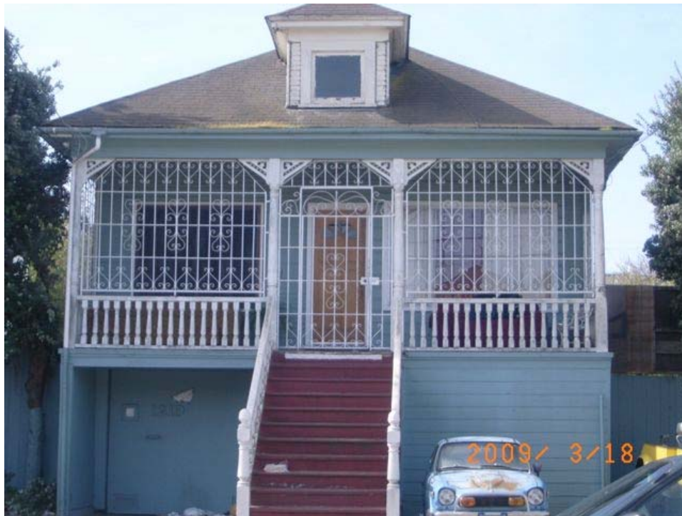
Hollister Avenue near Jennings Street: deteriorated roof, evidence of dry rot, peeling paint, security gate, apparently inoperable vehicle.
