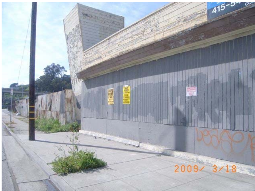
Industrial Street near Loomis Street: vacant and dilapidated building, peeling paint, dry rot, graffiti, security camera warning, informal and substandard construction of fence.
