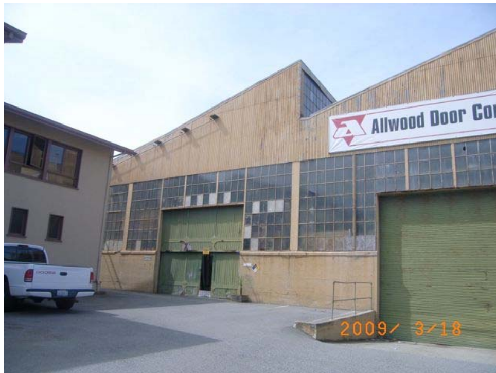
3 rd Street near Egbert Avenue: extensive deterioration rusted metal siding, peeling paint, broken windows.
