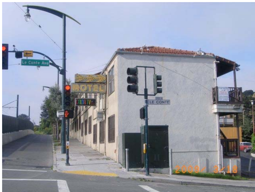
LeConte Avenue and 3 rd Street: motel property for sale exhibiting faded and peeling paint, cracked walls, extensive deferred maintenance, protective bars on windows.
