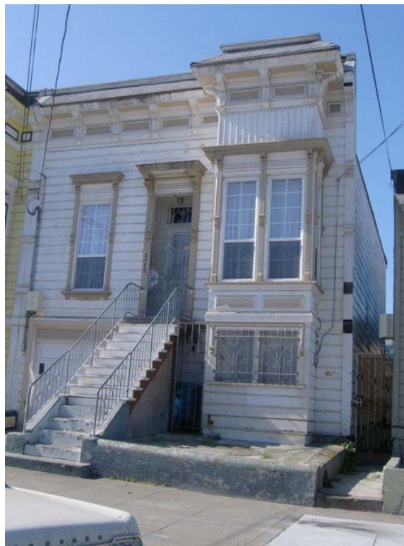
Newcomb Avenue near Newhall Street: peeling paint, water damage, evidence of dry rot.
