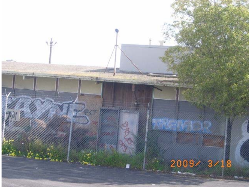
Cesar Chavez Street near I-280: vacant building, boarded windows, graffiti, extensive dilapidation, vegetation growing in rain gutters.
