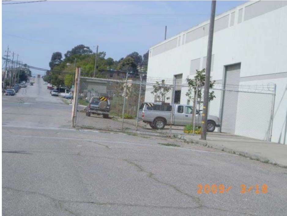
Palou Avenue near Griffith Street: fence blocking pedestrian access to public right-of-way.
