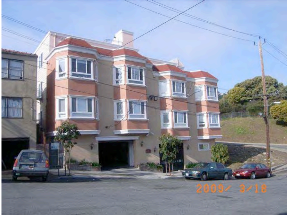
LeConte Avenue near 3 rd Street: new residential construction.
