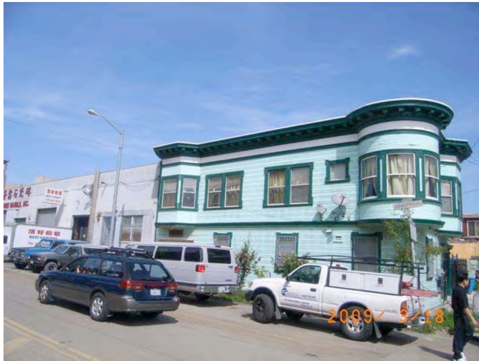
Armstrong Avenue at 3 rd Street: residential building abutting warehouse, evidence of incompatible uses.
