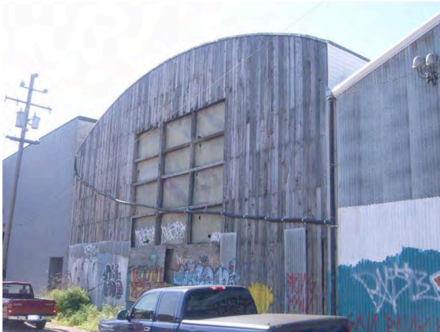
Newcomb Avenue near Toland Street: dilapidated building, graffiti, informal and substandard construction, broken windows.
