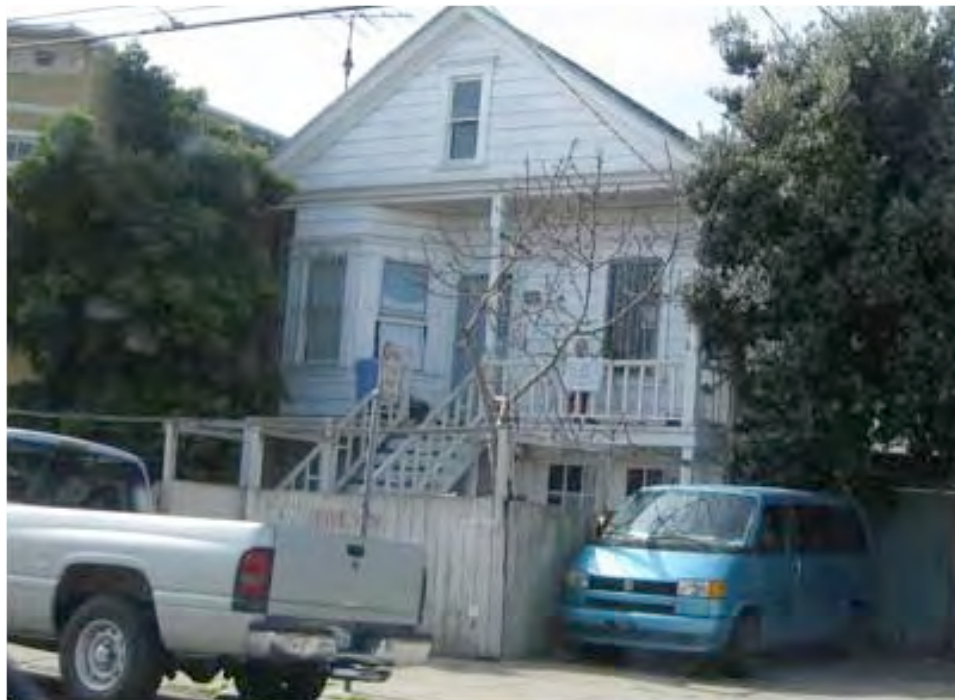
Hollister Avenue near Jennings Street: deteriorating fence, security door, security grates on windows.
