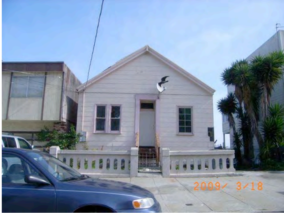
Ingerson Avenue near Hawes Street: deteriorated, missing siding, informal and substandard construction, broken window.
