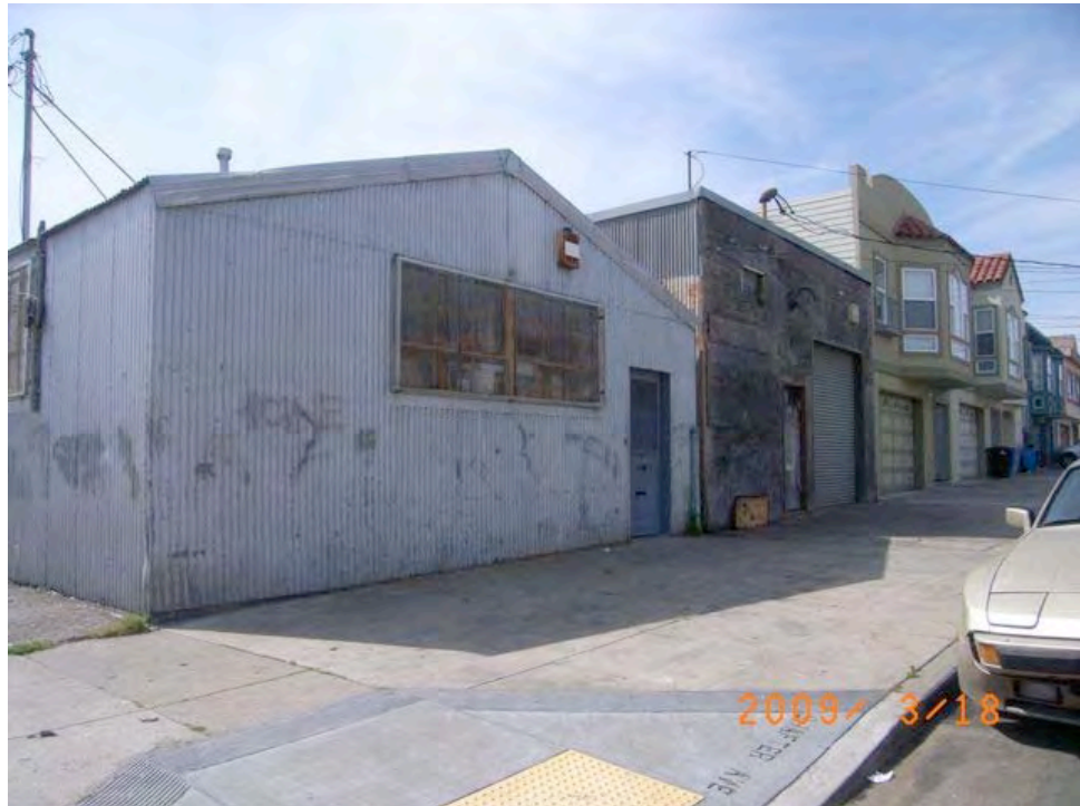
Shafter Avenue near Hawes Street: informal and substandard construction, dilapidated building, deteriorating siding, graffiti.
