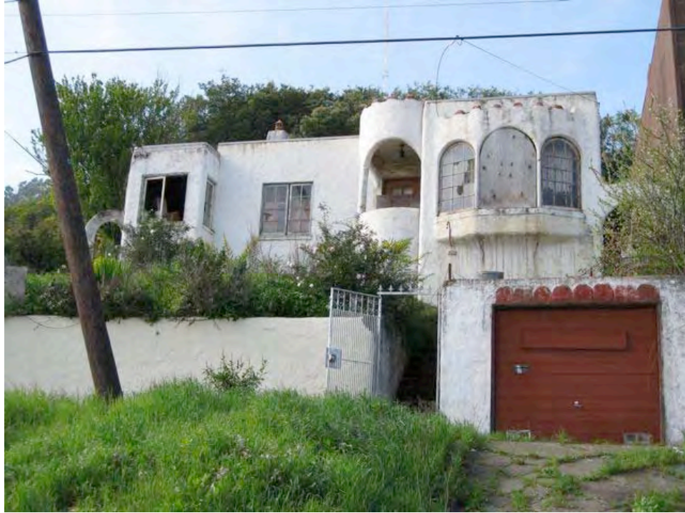
Jamestown Avenue near Redondo Street: vacant building, extensive dilapidation, broken and boarded windows, overgrown landscaping.
