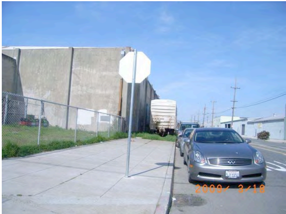
Carroll Avenue near Jennings Street: cracked concrete structure, graffiti removal, abandoned train car stored in public right-of-way, unpaved sidewalk.
