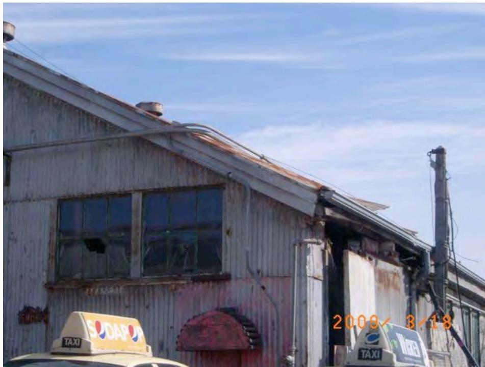
Marin Street near Jerrold Avenue: extensive dilapidation, informal and substandard construction, broken windows, graffiti, deteriorated roofing.
