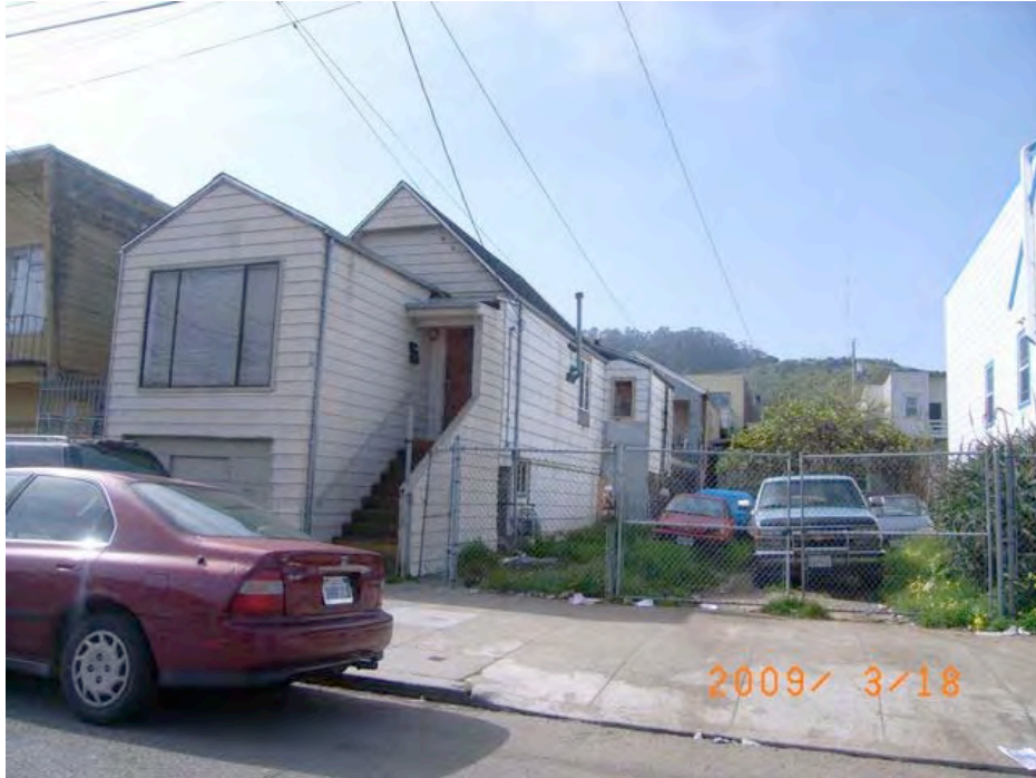
Fitzgerald Avenue near Ingalls Street: trash accumulation, vacant lot used as auto storage, peeling paint.
