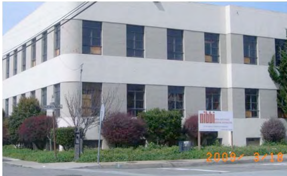
Egbert Avenue and Newhall Street: property with peeling paint and boarded windows.
