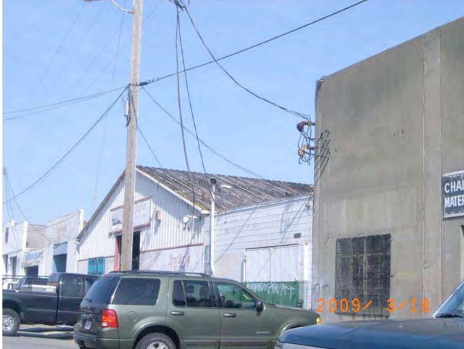
Egbert Avenue near Jennings Street: deteriorated metal roof, damaged siding, security grate, graffiti.
