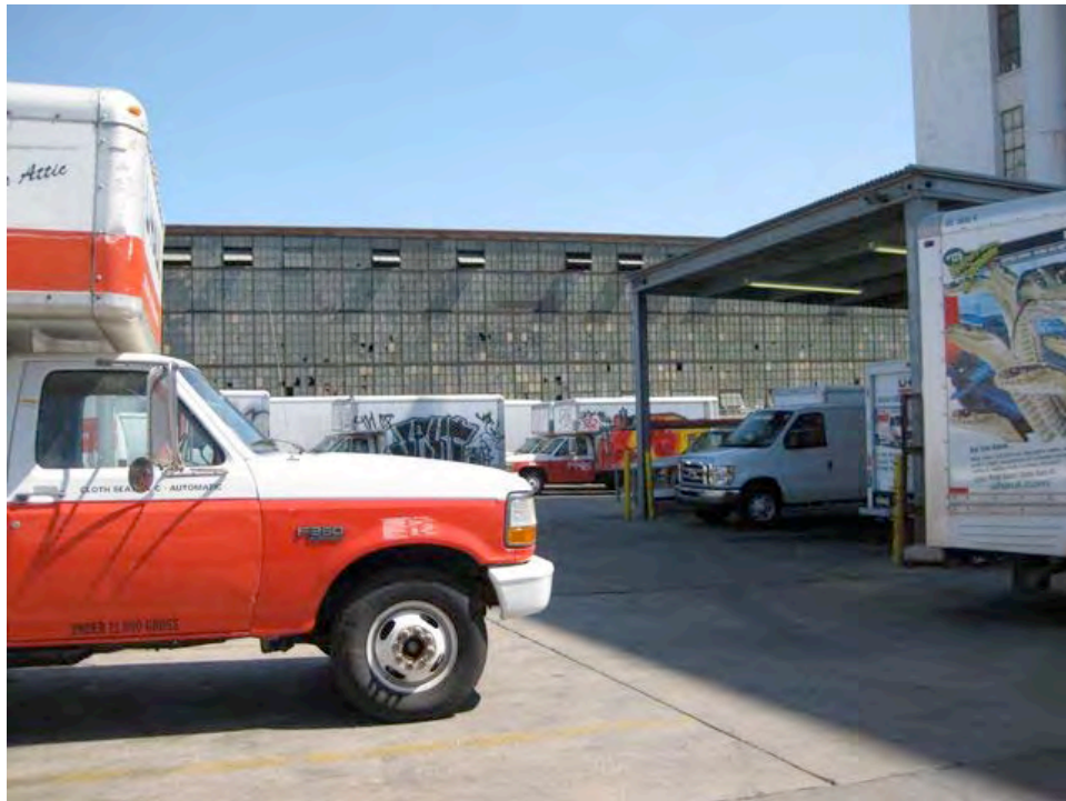
Near Bayshore Boulevard and Paul Avenue: apparently abandoned building, broken and boarded windows, graffiti.
