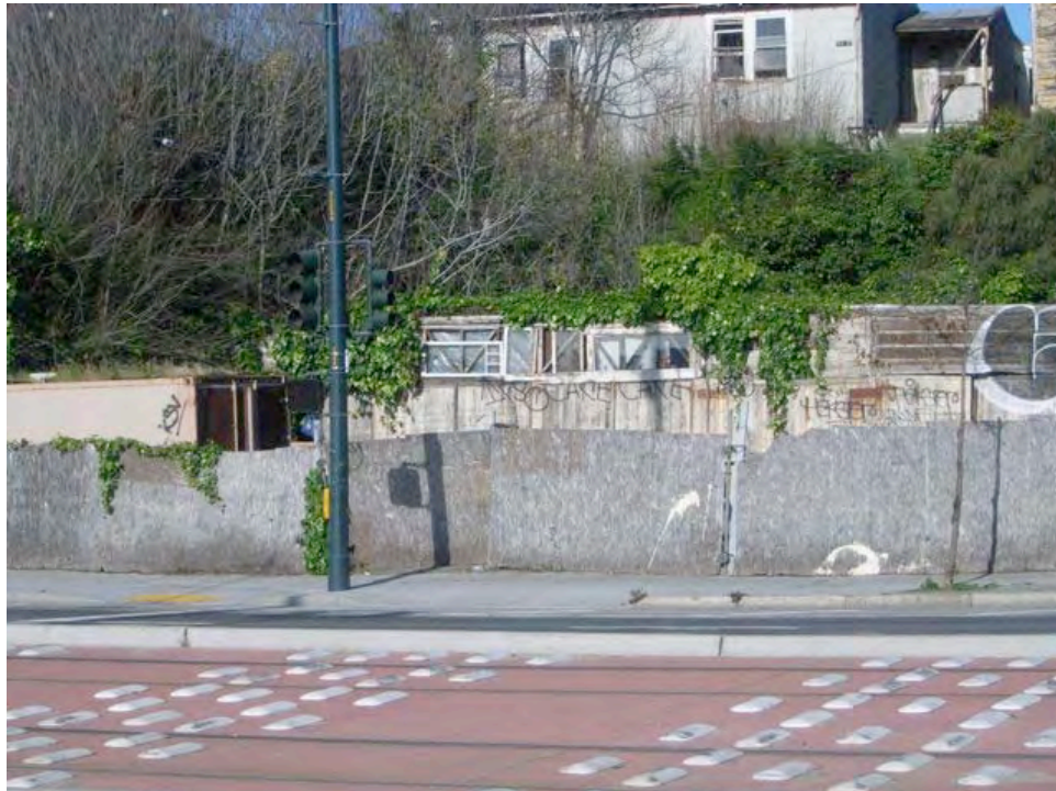
3 rd Street near Thornton Avenue: informal and substandard structure, graffiti, extensive dilapidation.
