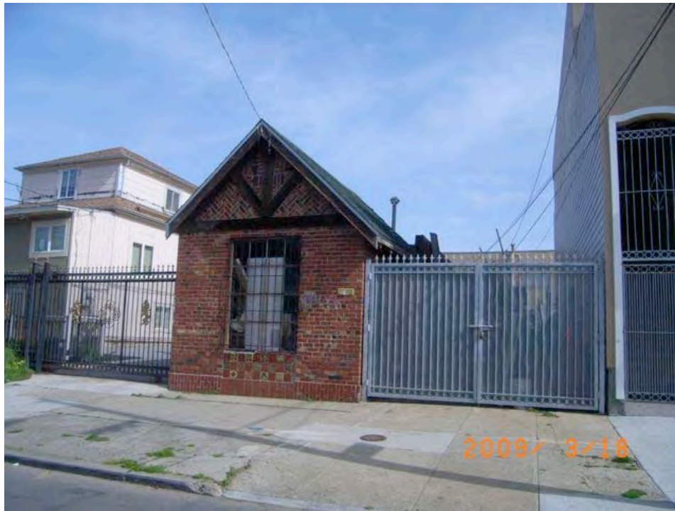
Fitzgerald Avenue near Hawes Street: unreinforced masonry construction, graffiti, security fencing.
