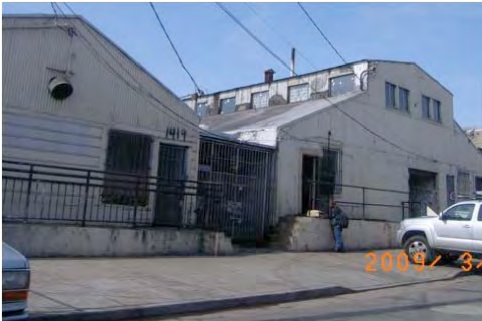
Egbert Avenue near Jennings Street: deteriorated roofing and siding, peeling paint, water damage.
