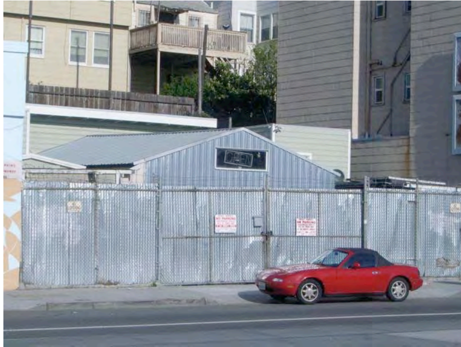
3 rd Street near Shafter Avenue: barbed wire, dented fencing, illegally parked car.
