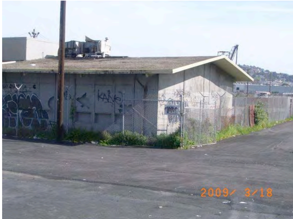
Cesar Chavez Street near I-280: graffiti, broken and boarded windows, barbed wire security fencing, extensive dilapidation.
