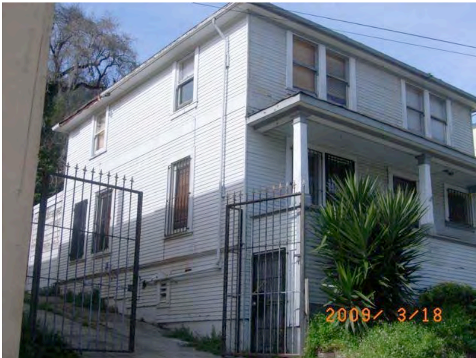
Ignacio Avenue near Ingerson Avenue: deteriorated siding, damaged gutters, peeling paint, security grates.
