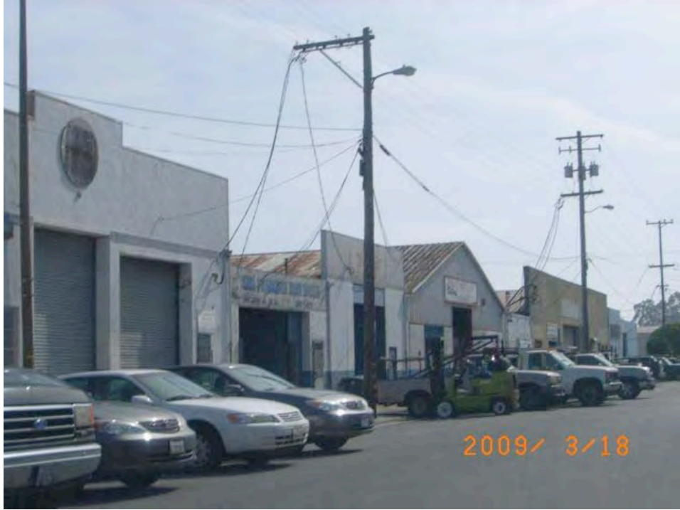
Egbert Avenue near 3 rd Street: roofing deterioration from rust.
