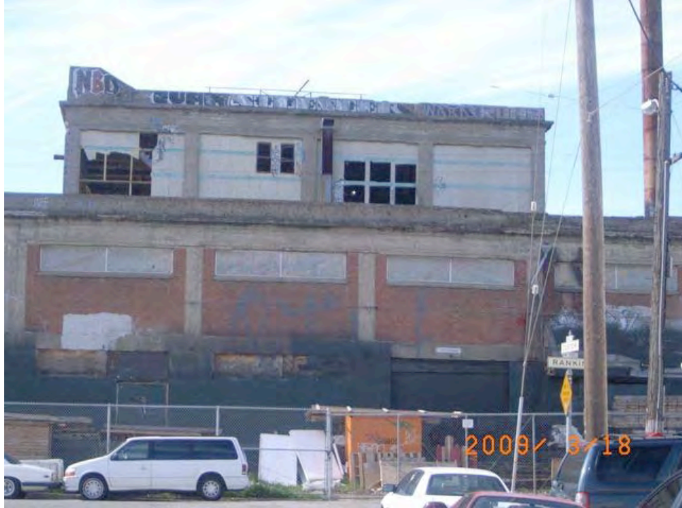
Custer Avenue near Rankin Street: abandoned building, cracked wall, fire damage, broken windows, extensive dilapidation, outdoor storage, graffiti.
