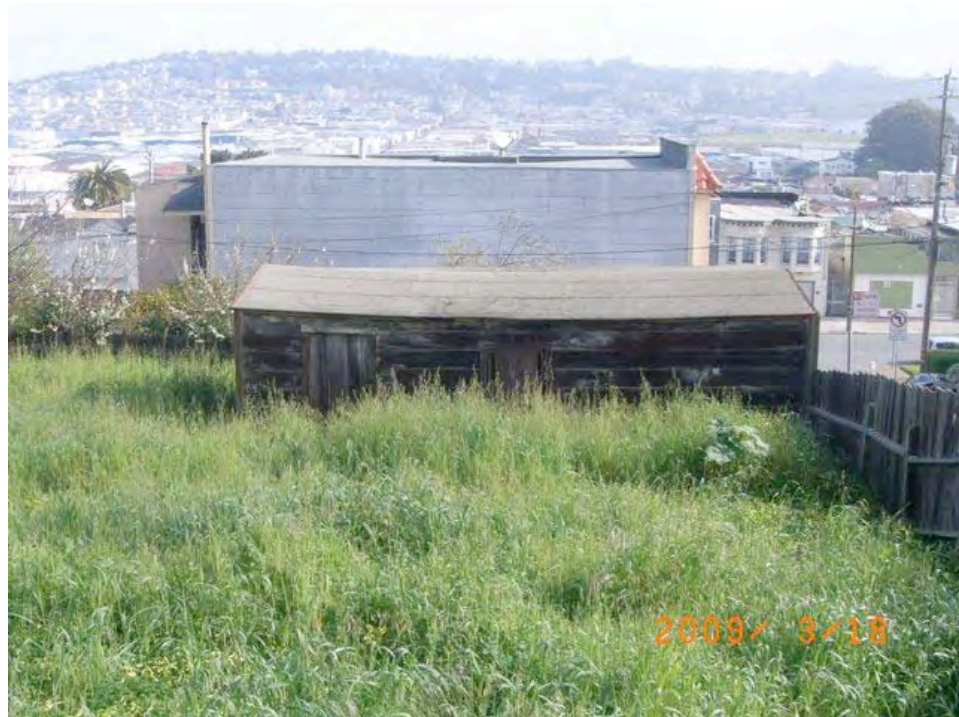
Redondo Street near Jamestown Avenue: extensive deterioration, sagging roof, peeling paint, overgrown landscaping, water damage.
