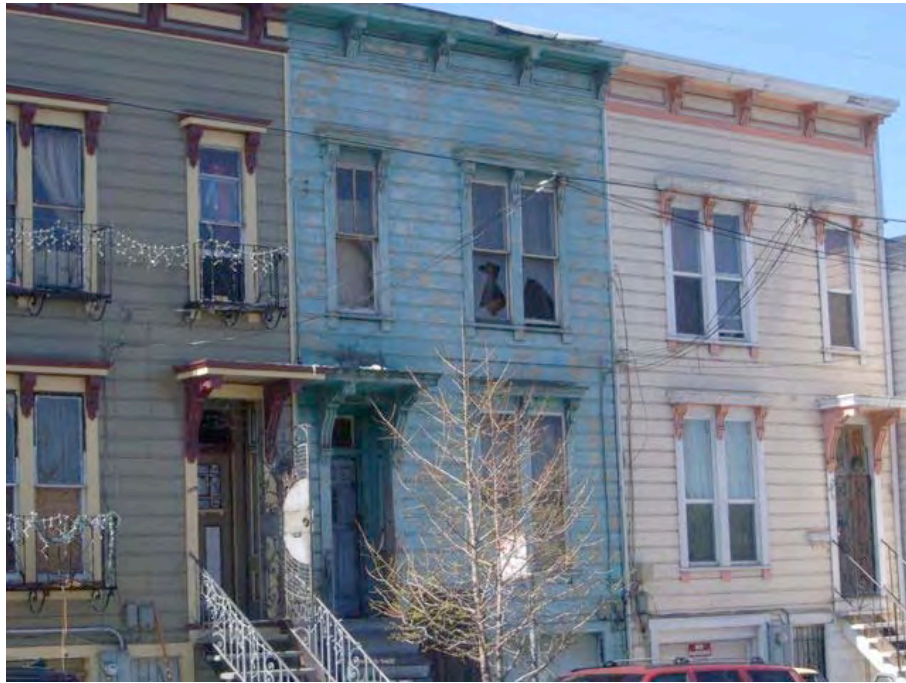
Oakdale Avenue near Quint Street: extensive dilapidation (middle building), broken windows, damaged eaves, broken and boarded windows.
