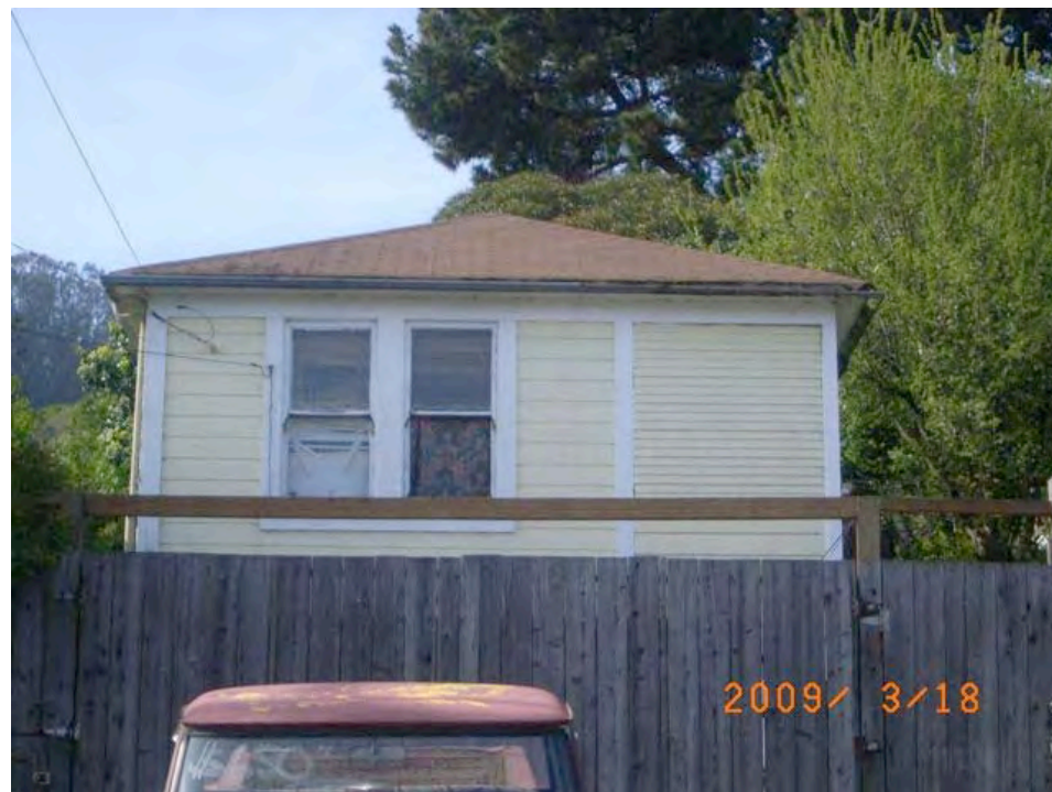
Ingerson Avenue near Redondo Street: peeling paint, deteriorated windows, abandoned vehicle.
