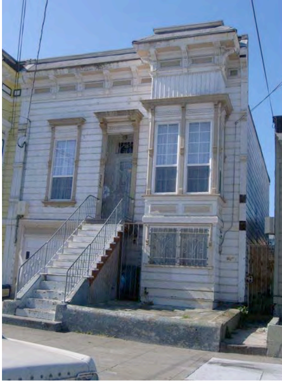
Newcomb Avenue near Newhall Street: peeling paint, water damage, evidence of dry rot.
