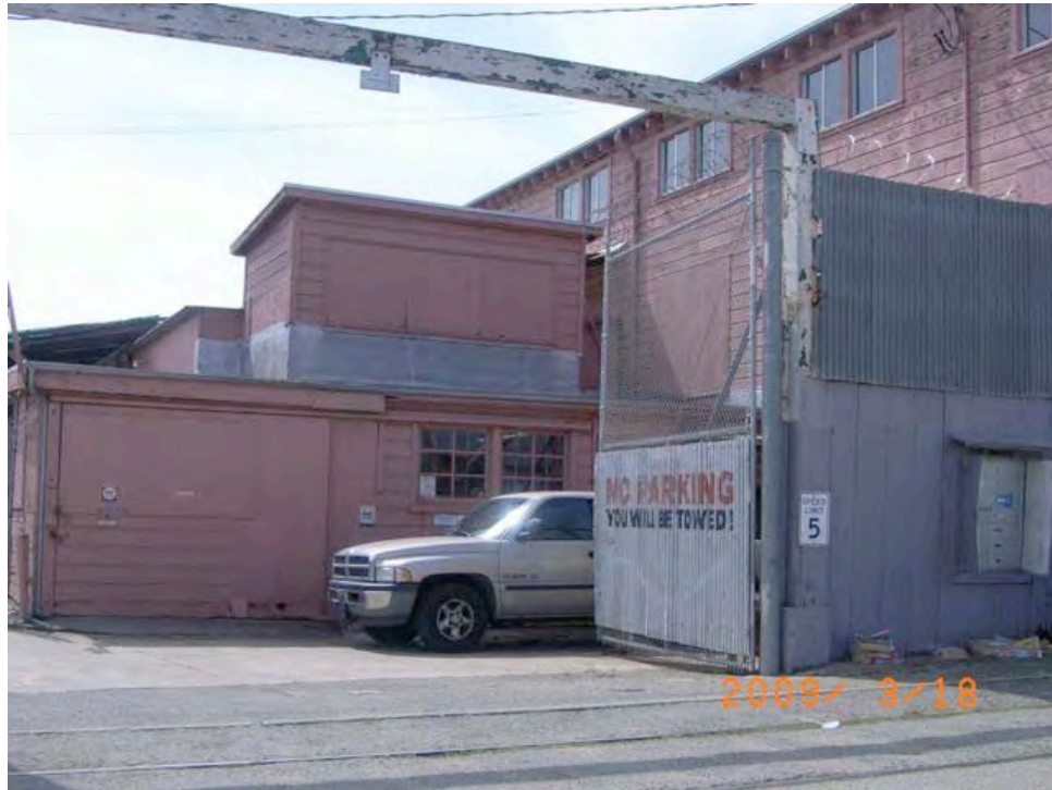
Egbert Avenue near Newhall Street: peeling paint; evidence of water damage; trash accumulation; lack of sidewalk, curb or gutter; and abandoned rail lines.
