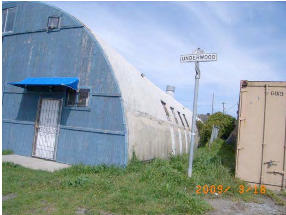
Underwood Avenue near Hawes Street: peeling paint; deteriorating siding, roofing and fencing; lack of sidewalk.
