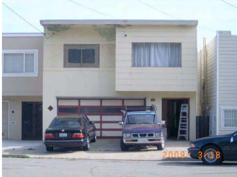
Jamestown Avenue near Griffith Street: peeling paint, deferred maintenance, water damage.
