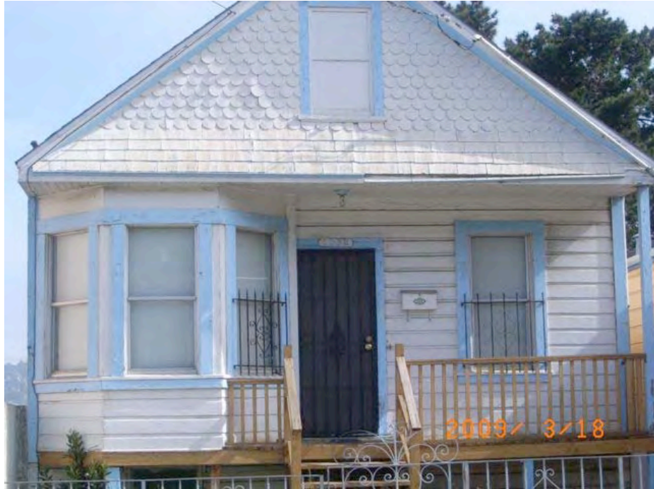
Hollister Avenue near Ingalls Street: deteriorated siding, security door, peeling paint, missing cripple wall.
