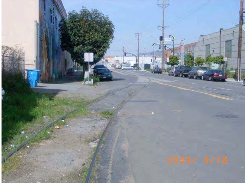
Carroll Avenue near Keith Street: abandoned train tracks, poor pedestrian access, incomplete sidewalk, overgrown landscaping.
