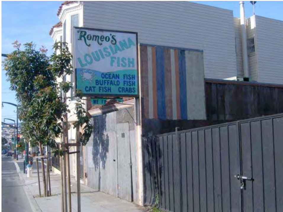
3 rd Street near Williams Avenue: abandoned business space, boarded storefront, extensive deterioration, informal and substandard construction.
