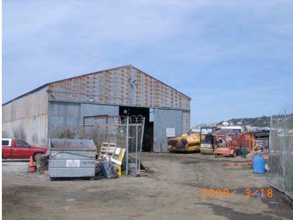
Armstrong Avenue at Griffith Street: rusted and deteriorated siding, outdoor storage, lack of sidewalks.
