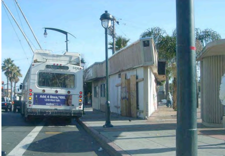
3rd Street near Palou Avenue: boarded door, graffiti, extensive deferred maintenance, alignment problems.
