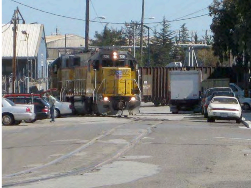
Quint Street near Davidson Avenue: lack of buffering between rail line and street, lack of pedestrian infrastructure, dilapidated pavement.
