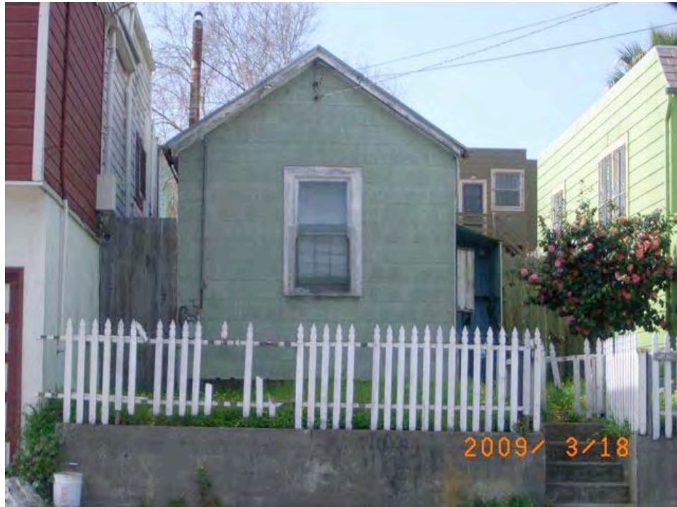
Gilman Avenue near Jennings Street: extensive deferred maintenance, peeling paint, deteriorating siding, broken eaves, cracked retaining wall, dilapidated fence.
