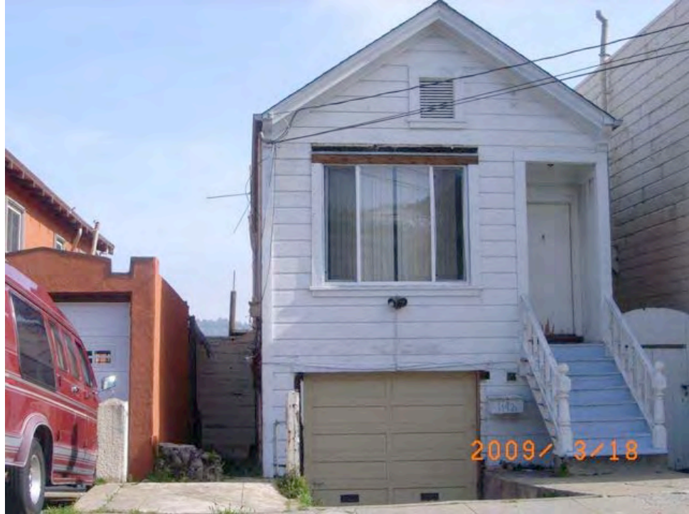
Hollister Avenue near Ingalls Street: extensive deterioration, deteriorated siding, external wiring, dilapidated door.
