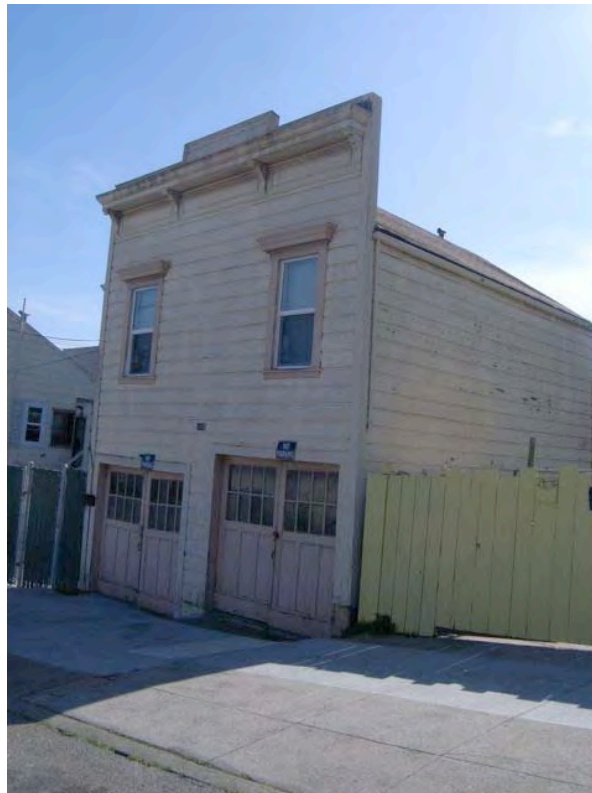
Phelps Street near Palou Avenue: deteriorated building, rotting garage door and peeling paint.
