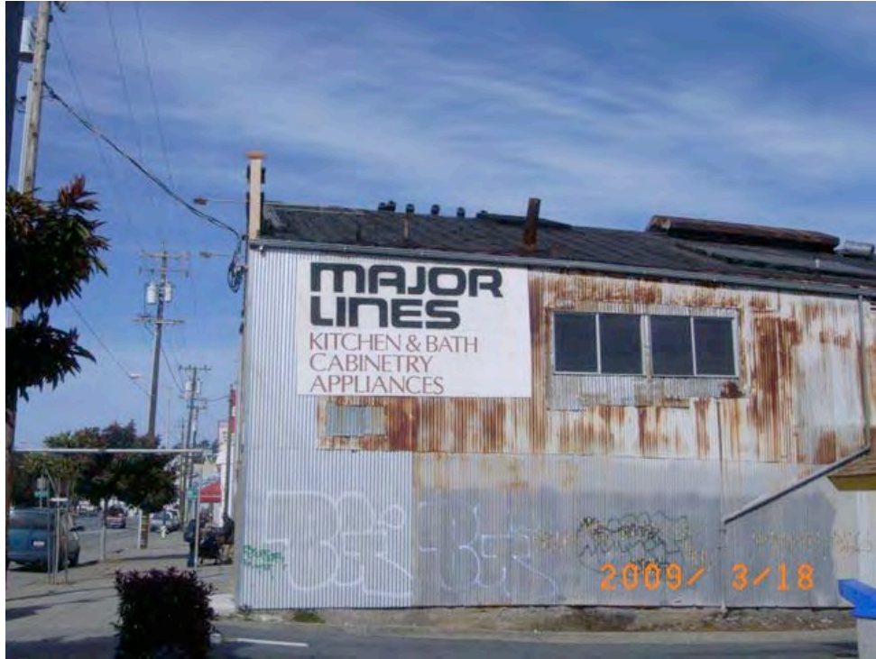
Bayshore Boulevard near Costa Street: eroded foundation, rusted and deteriorated siding, damaged roof, extensive deterioration, informal and substandard construction.
