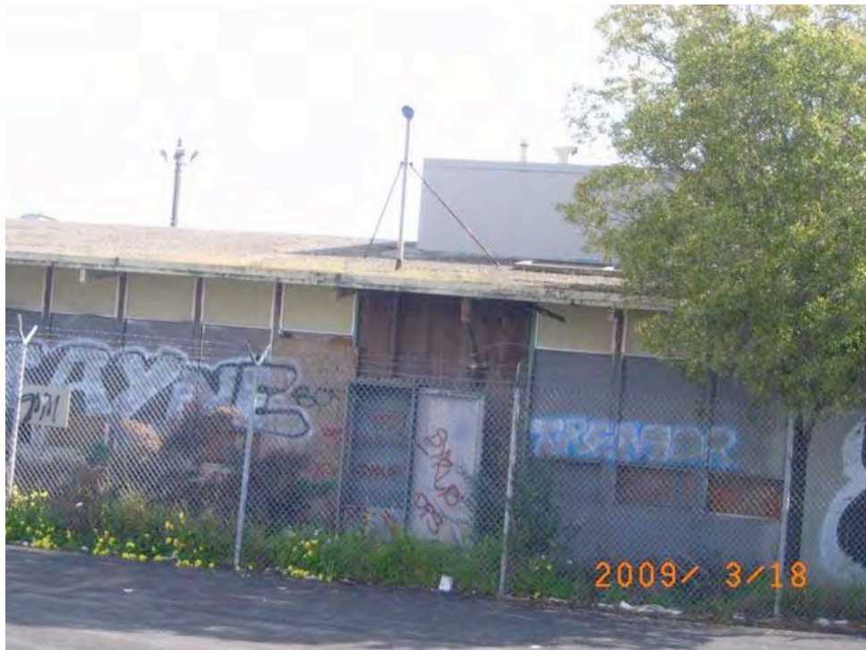
Cesar Chavez Street near I-280: vacant building, boarded windows, graffiti, extensive dilapidation, vegetation growing in rain gutters.
