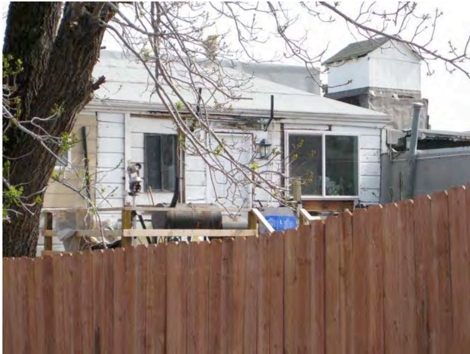
Hollister Avenue near Hawes Street: peeling paint, dry rot, cracked siding, informal and substandard construction.
