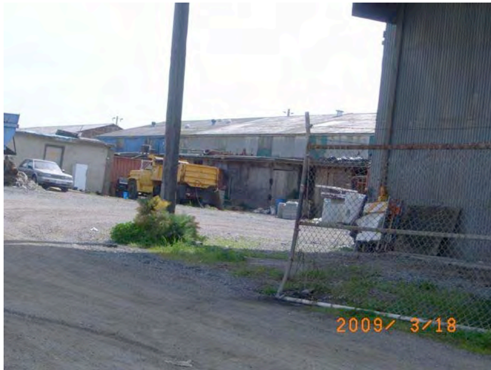
Yosemite Avenue near Hawes Street: deteriorated buildings, outdoor storage, informal and substandard construction.
