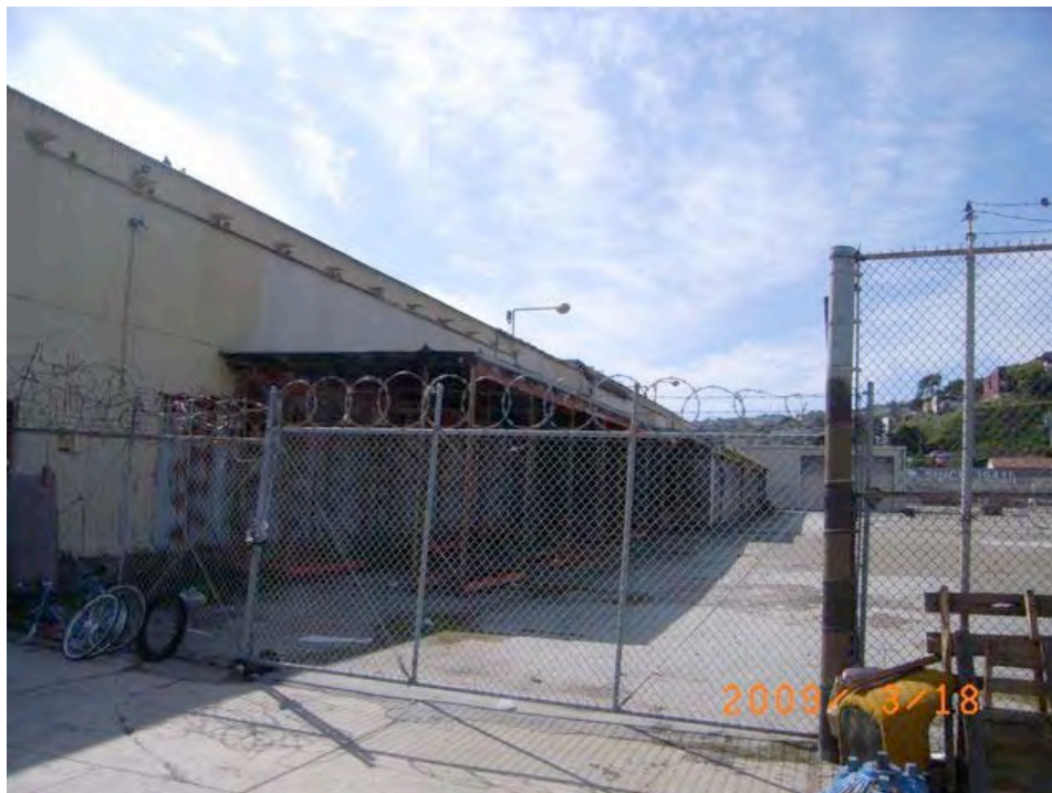
Loomis Street near Waterloo Street: vacant warehouse space, outdoor storage, trash dumping, razor wire security fencing.
