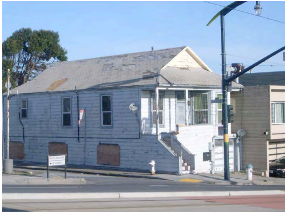
3 rd Street at Salinas Avenue: extensive dilapidation, peeling paint, boarded windows, deteriorating roofing and eaves.
