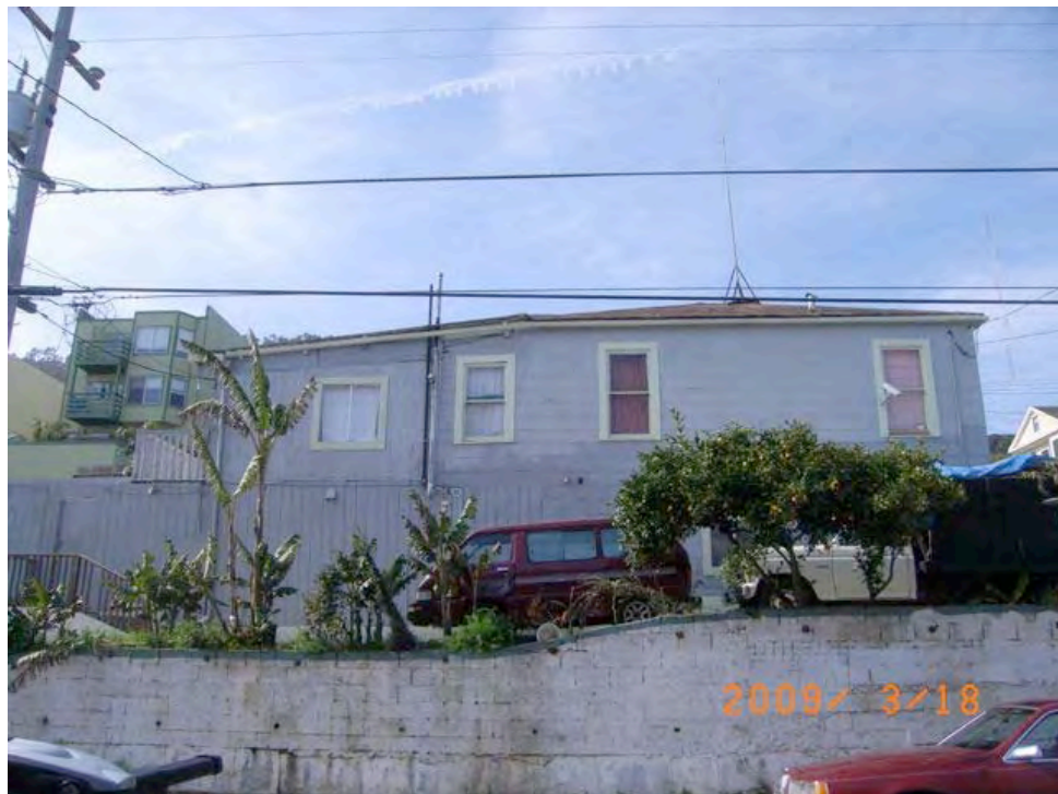
Ingerson Avenue near Hawes Street: aging retaining wall supporting driveway, residence with faded paint, water damage, security camera.
