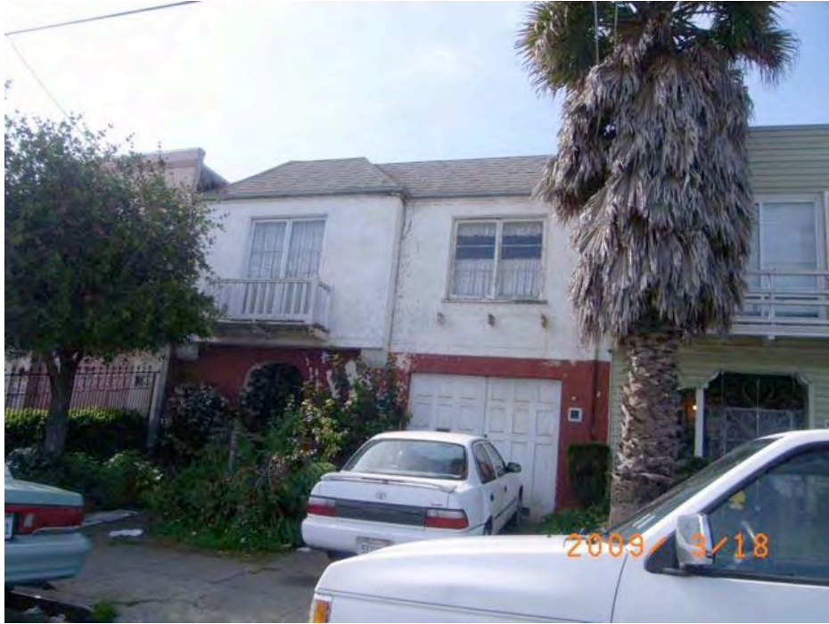
Fitzgerald Avenue near Jennings Street: deferred maintenance, evidence of dry rot, peeling paint.
