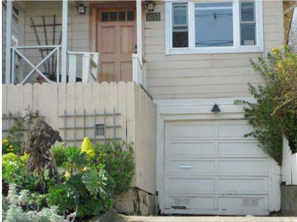
Ingerson Avenue near Ingalls Street: foundation and frame damage, evidence of dry rot.
