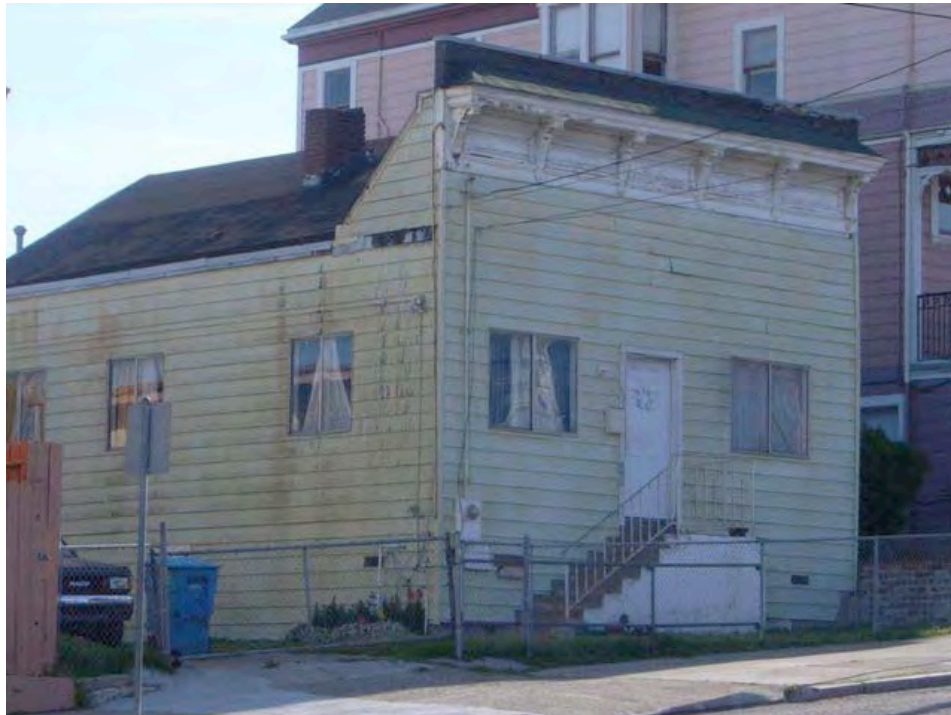
3rd Street near Jerrold Avenue: extensive deterioration, peeling paint, water damage, deteriorating roof and chimney.
