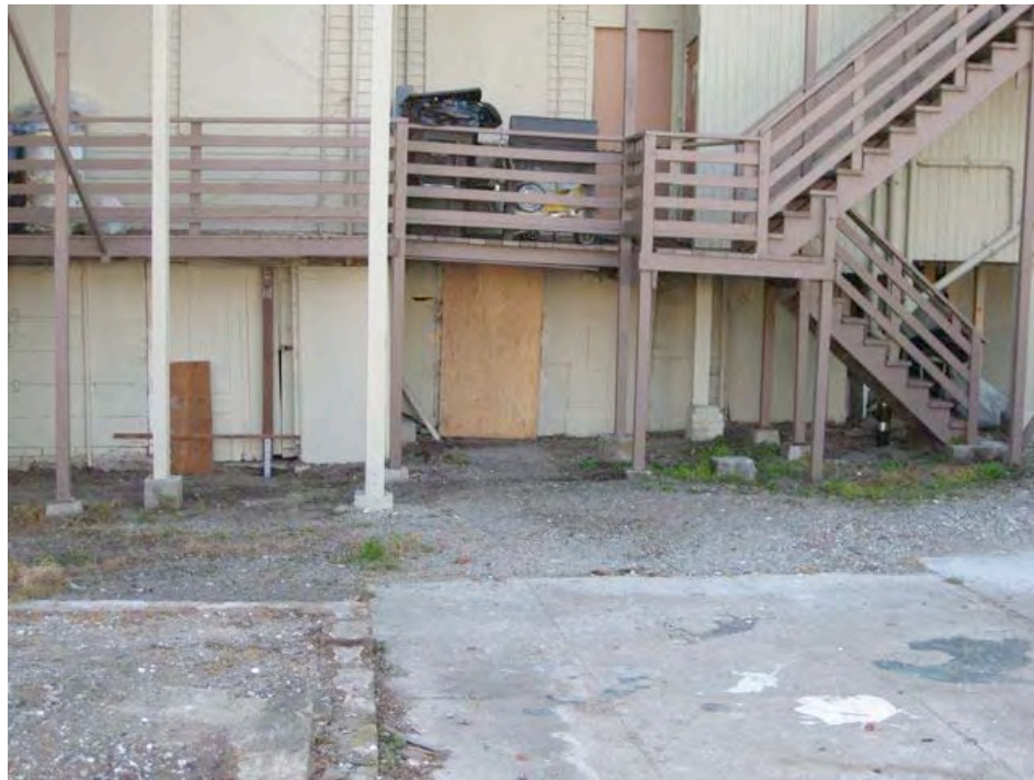
Newhall Street near Lasalle Avenue: informal and substandard construction, alignment problems, boarded doors.
