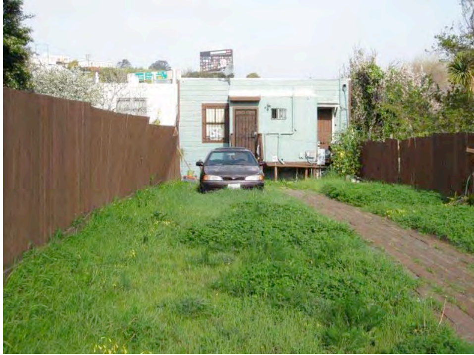
3 rd Street near Key Avenue: informal and substandard construction, extensive deterioration.
