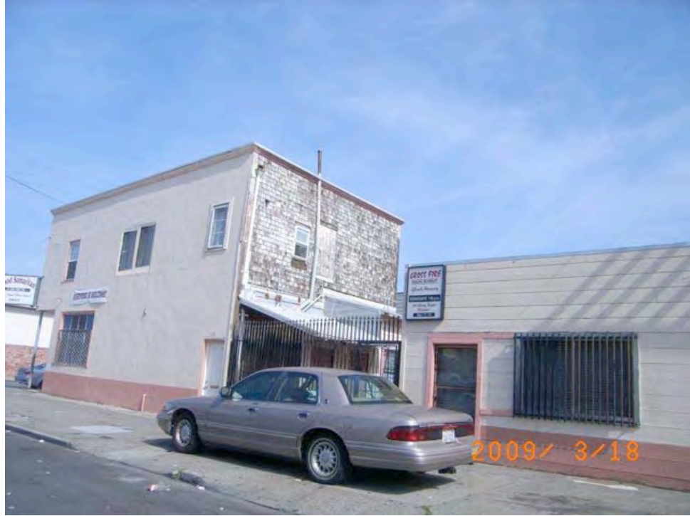
Fitzgerald Avenue near Ingalls Street: security grates, deteriorated siding, peeling paint.
