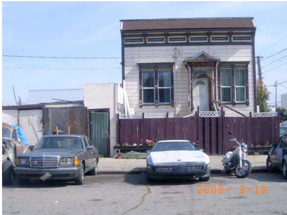
Egbert Avenue near Ingalls Street: informal and substandard construction, water damage, outdoor storage.
