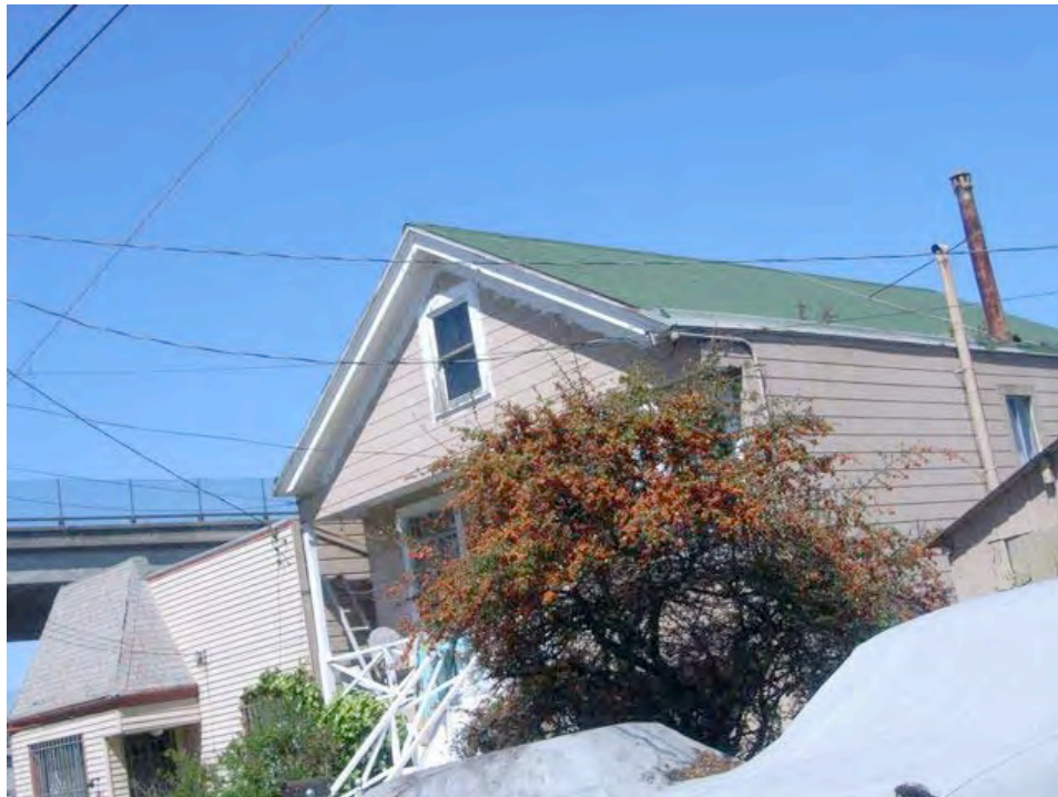
Revere Avenue near I-280: deteriorated building, lack of highway buffer, vegetation growing in gutter, peeling paint.
