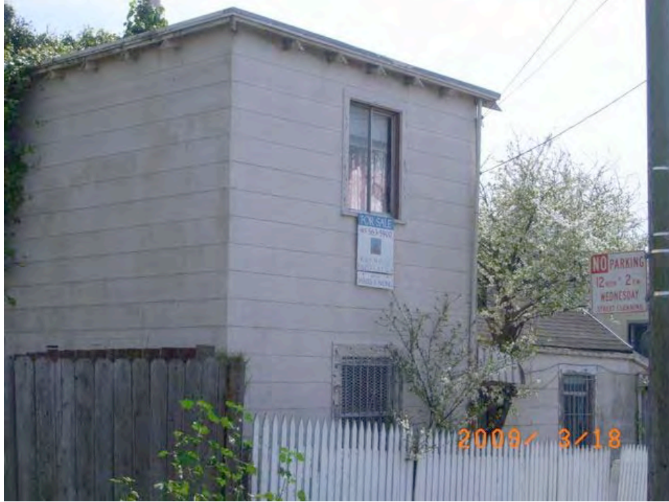
Keith Street near Underwood Avenue: peeling paint, sagging roof, dry rot, extensive deterioration of smaller building, missing eaves.
