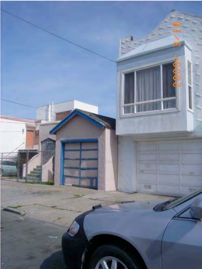
Fitzgerald Avenue near Hawes Street: deteriorated roofing, extensive deferred maintenance, dilapidated garage door.
