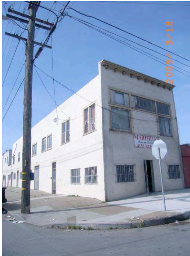
Egbert Avenue and Jennings Street: deteriorated, broken and boarded windows, informal external wiring, peeling paint.
