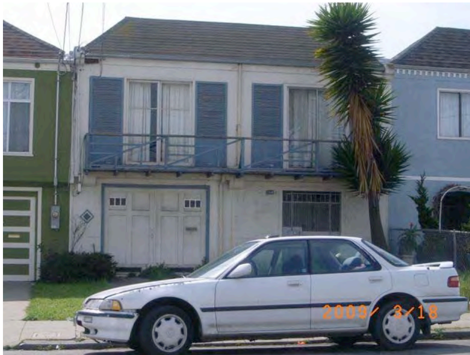
Wallace Avenue near Keith Street: deteriorated building, peeling paint, dry rot.
