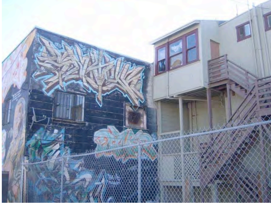
Newhall Street near Lasalle Avenue: alignment problems, substandard construction, broken and boarded windows.
