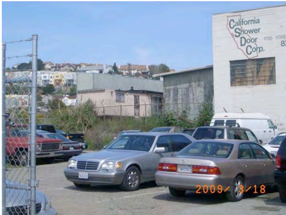
Armstrong Avenue near Mendell Street: peeling paint and deteriorated doors and windows. Shed shows signs of water damage and rotting wood.
