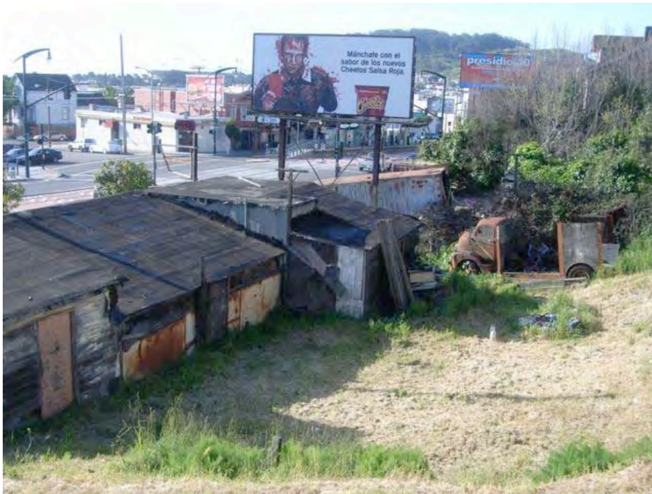
3 rd Street at Thornton Avenue, rear: extensive dilapidation, deteriorating roof and walls, substandard and informal construction, outdoor trash dumping.
