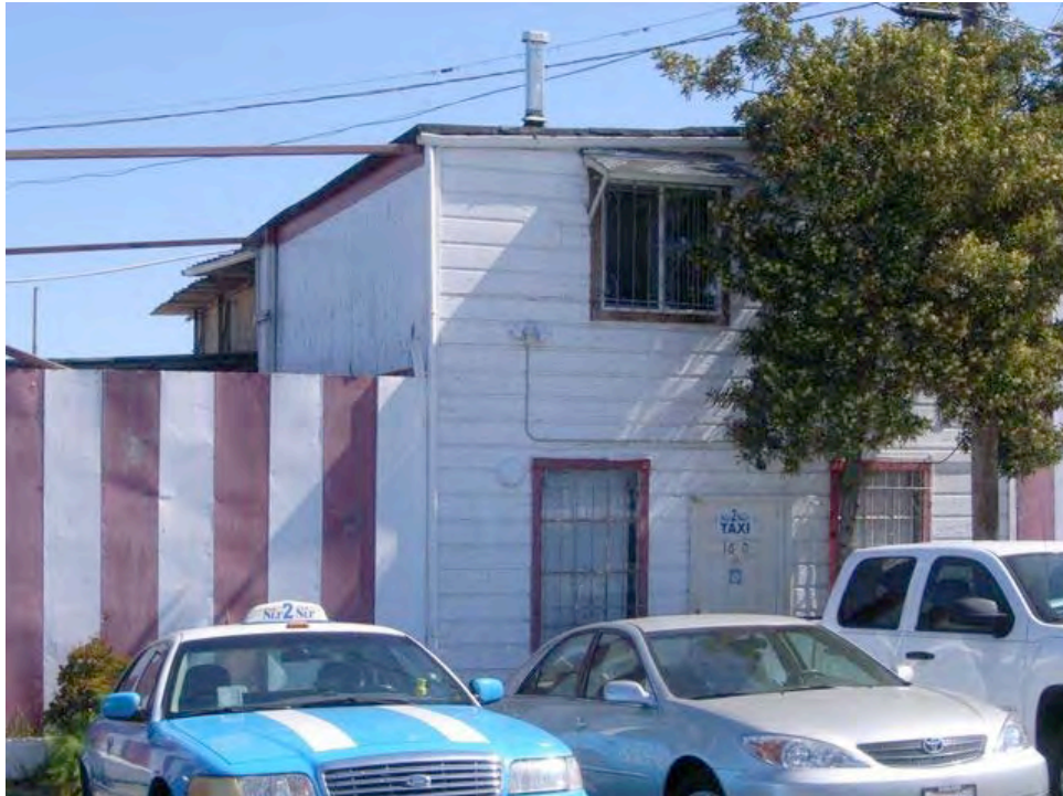
Davidson Avenue near I-280: extensive deferred maintenance, peeling paint.
