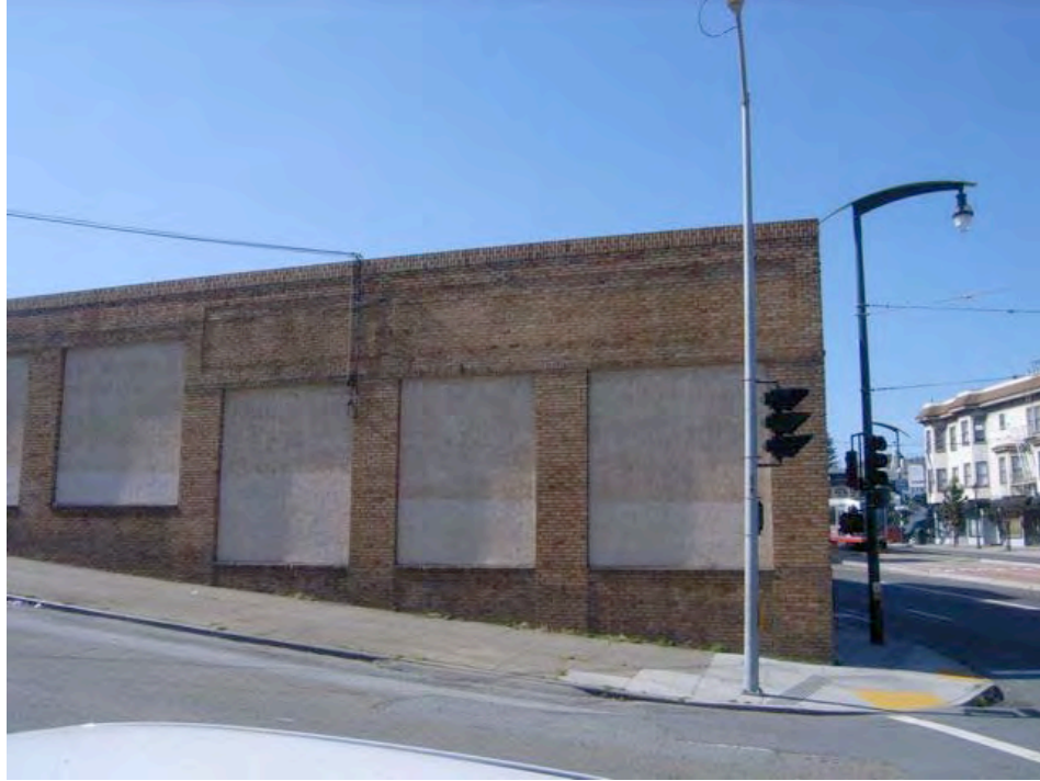
3 rd Street at Jerrold Avenue: vacant commercial building, partially reinforced masonry construction, boarded windows.
