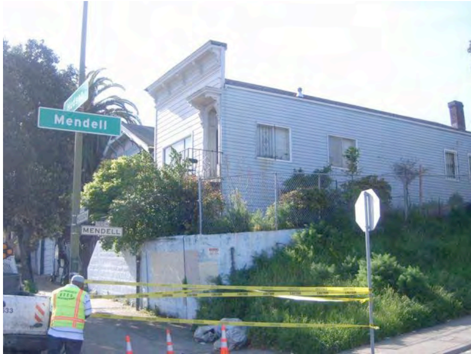
Hudson Avenue at Mendell Street: cracked and leaning retaining wall, extensive deterioration, water damage, boarded window.
