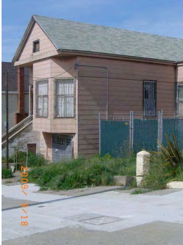
Newcomb Avenue near Lane Street: water damage, faded paint, deteriorated fencing, overgrown landscaping.
