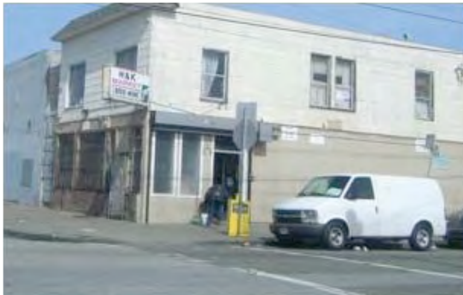
Fitzgerald Avenue near Jennings Street: liquor store with security grates, dilapidated siding.
