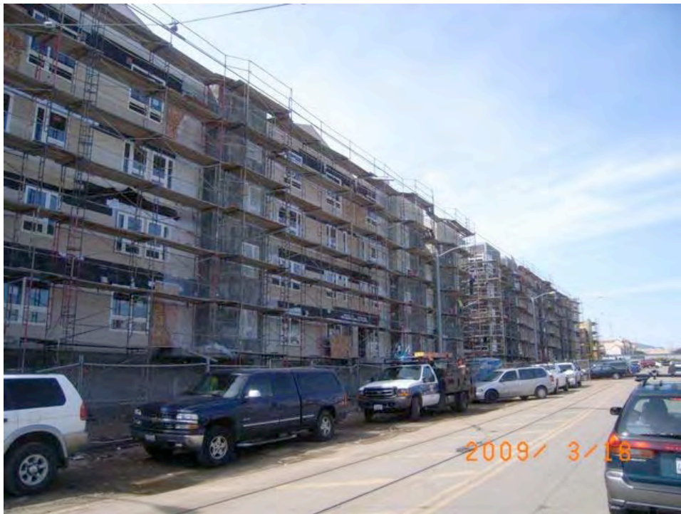
Armstrong Avenue near 3 rd Street: new housing construction.
