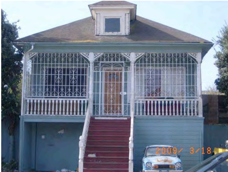
Hollister Avenue near Jennings Street: deteriorated roof, evidence of dry rot, peeling paint, security gate, apparently inoperable vehicle.
