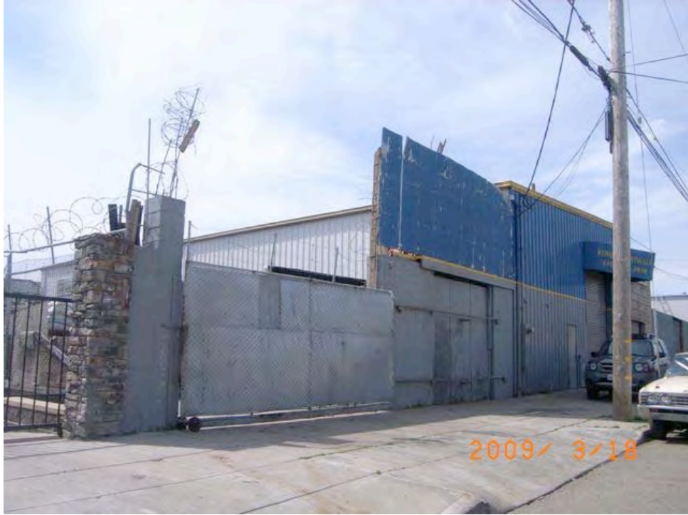
Thomas Avenue near Ingalls Street: severely deteriorated façade, informal and substandard construction, peeling paint, razor wire security fence.
