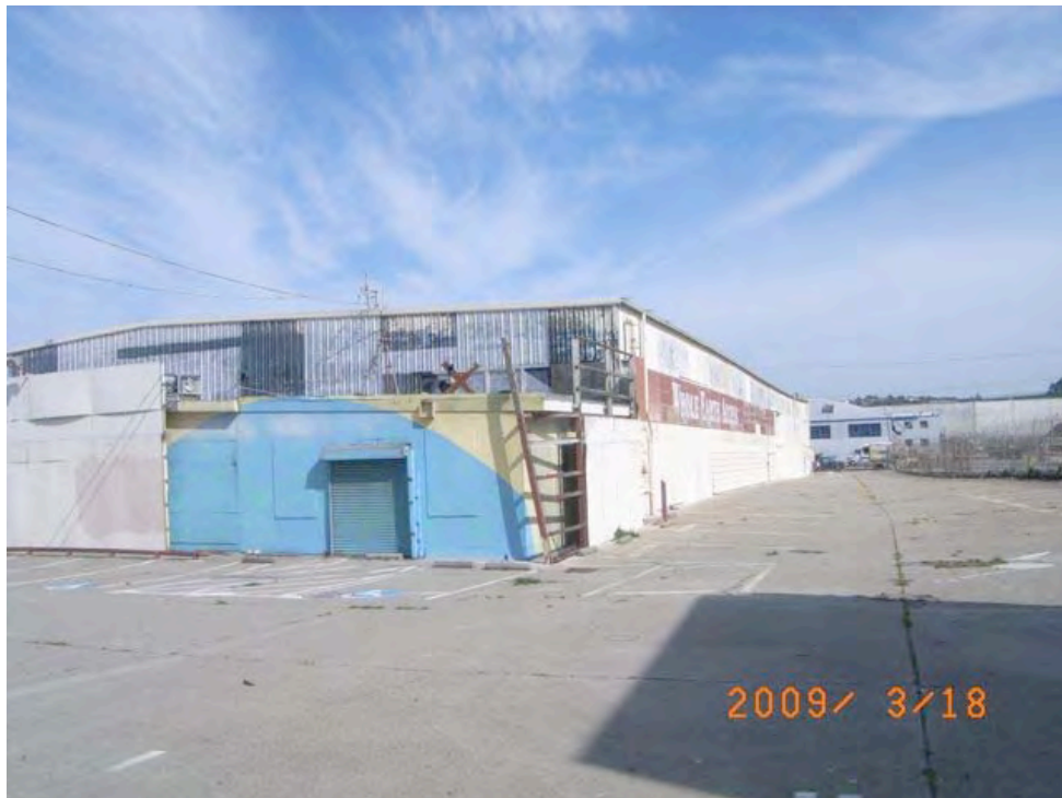
Bayshore Boulevard near Cortland Avenue: vacant building, informal and substandard construction, extensive deterioration, peeling paint.
