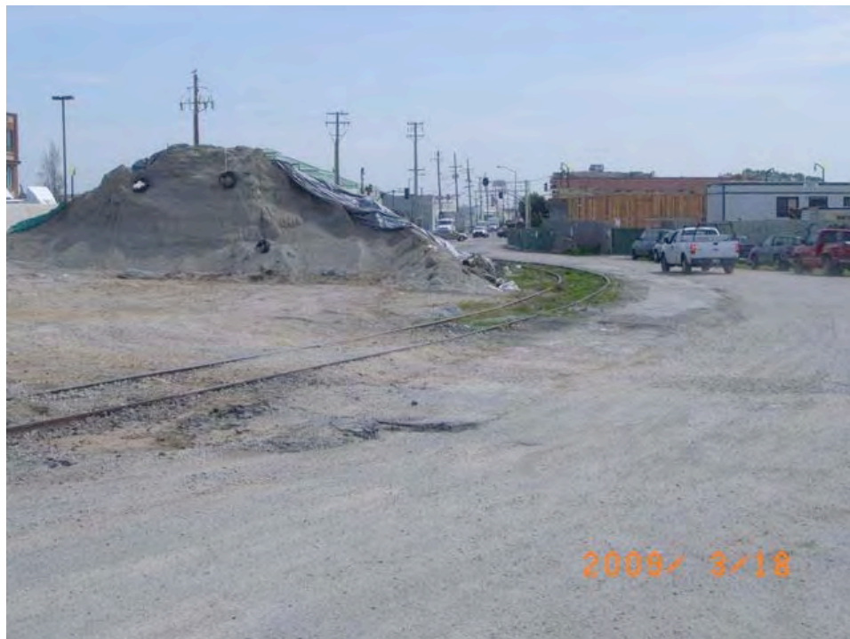
Carroll Avenue near Mendell Street: lack of sidewalk, curb or gutter; inadequate public improvements; open gravel pile; and abandoned train tracks.
