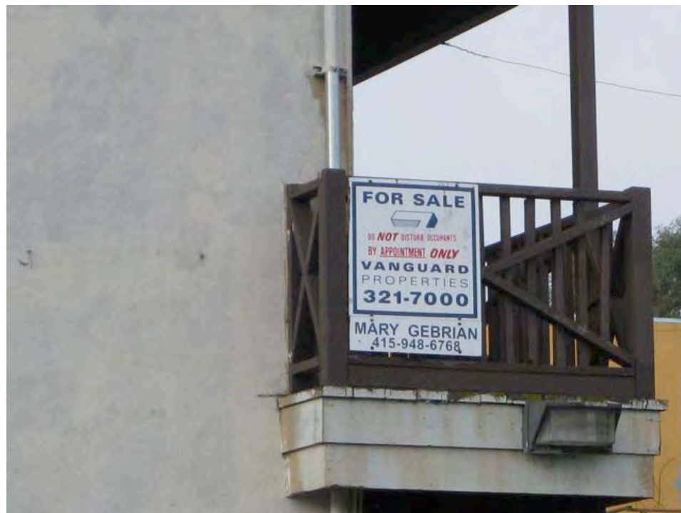
LeConte Avenue and 3 rd Street (close up of above): faded paint and water damage on walls.
